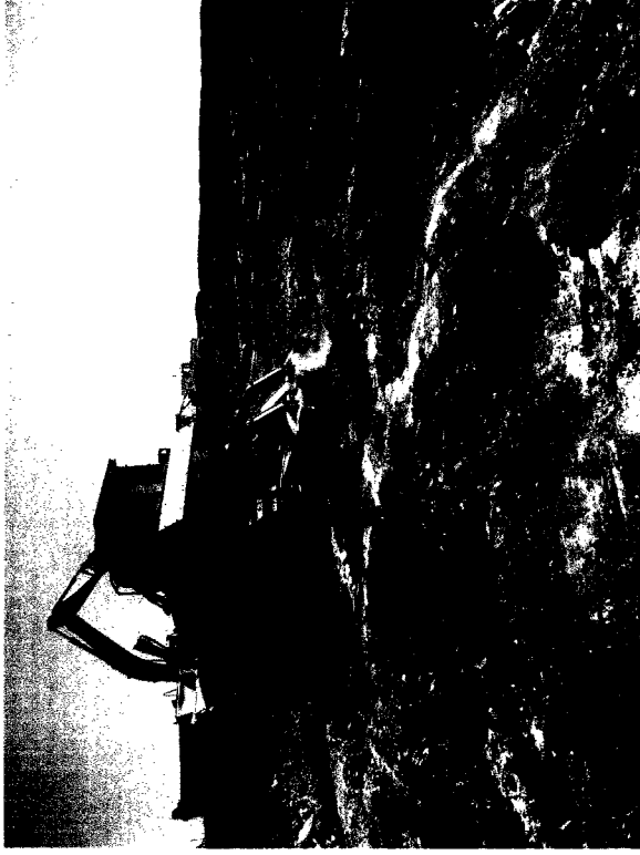
Ripping Rock with Dozer
