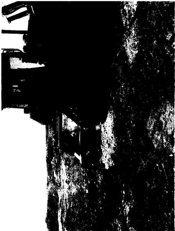
Ripping Rock with Dozer
