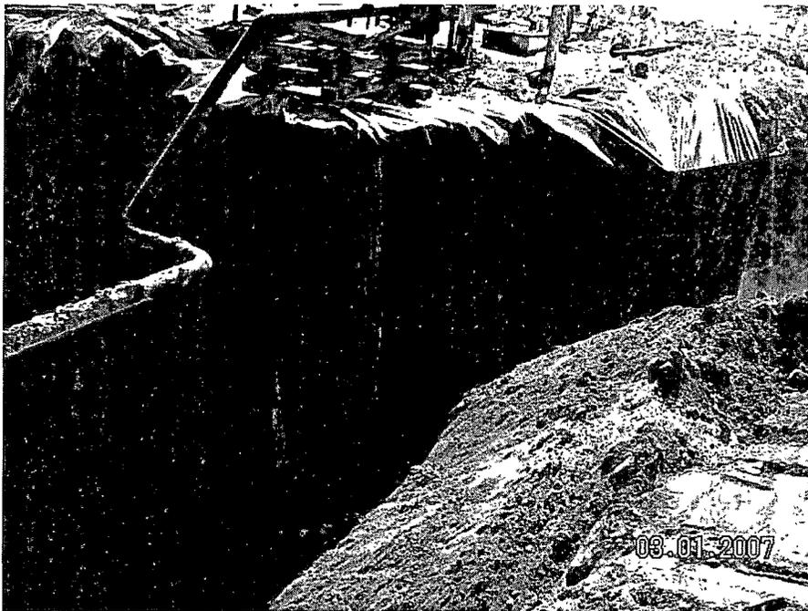
*Photo #6:* Looking southeasterly across excavation at installation of impermeable barrier.
