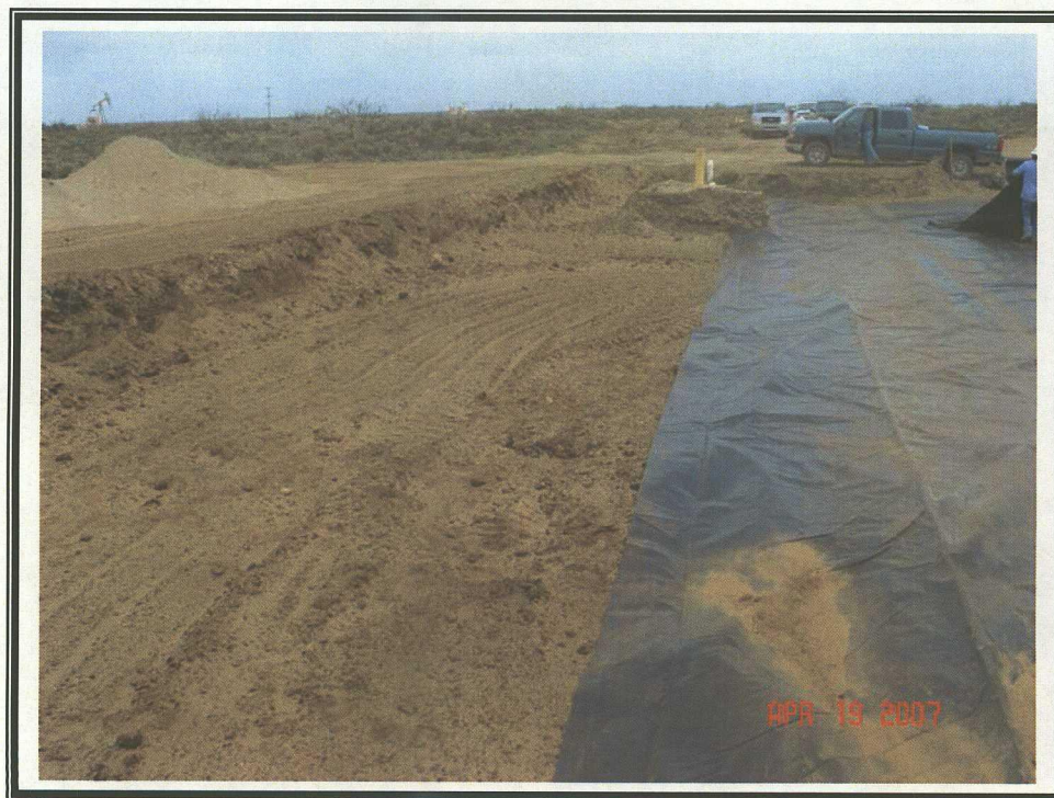
Installation of 20 mil Plastic Liner – MW-1 Area
