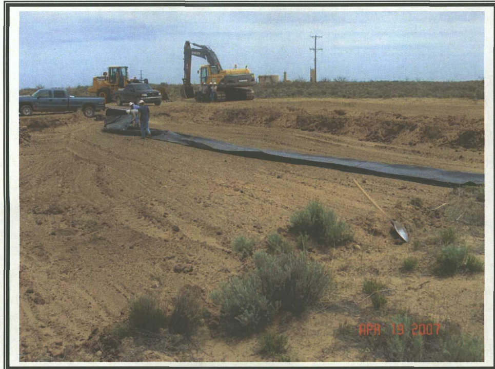
Installation of 20 mil Plastic Liner – MW-1 Area
