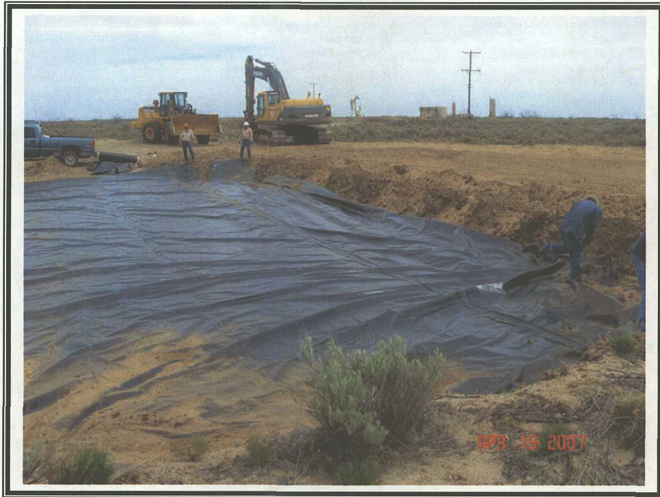
Installation of 20 mil Plastic Liner – MW-1 Area
