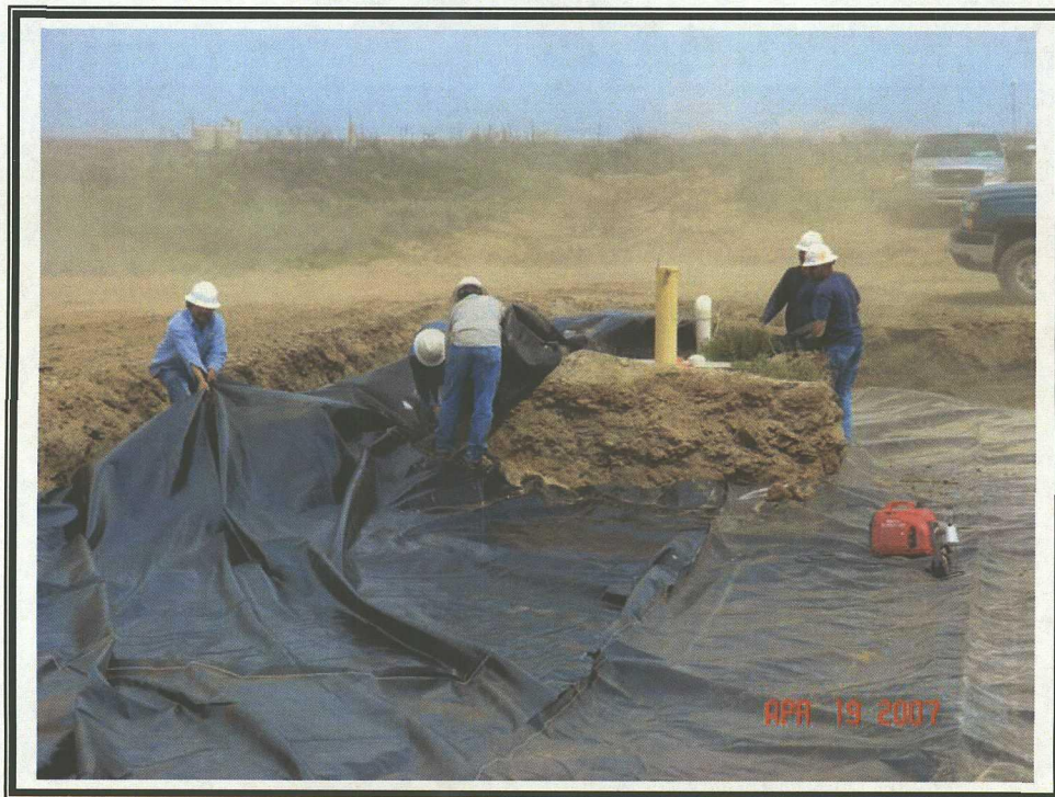
Installation of 20 mil Plastic Liner – MW-1 Area
