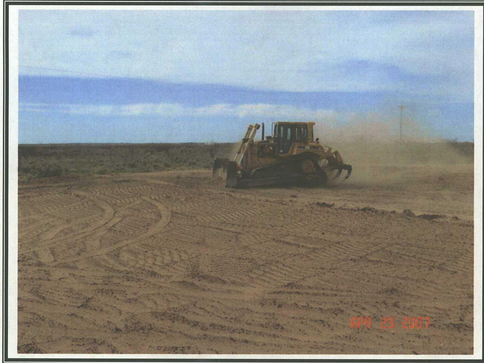
Site Backfilling
