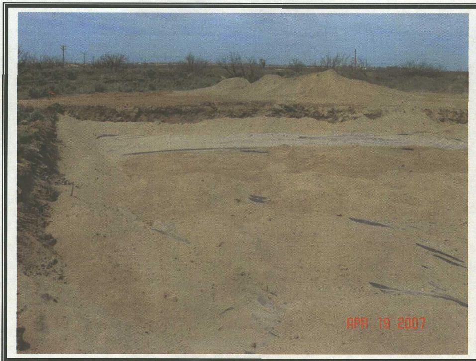
Backfilling of MW-1 Area
