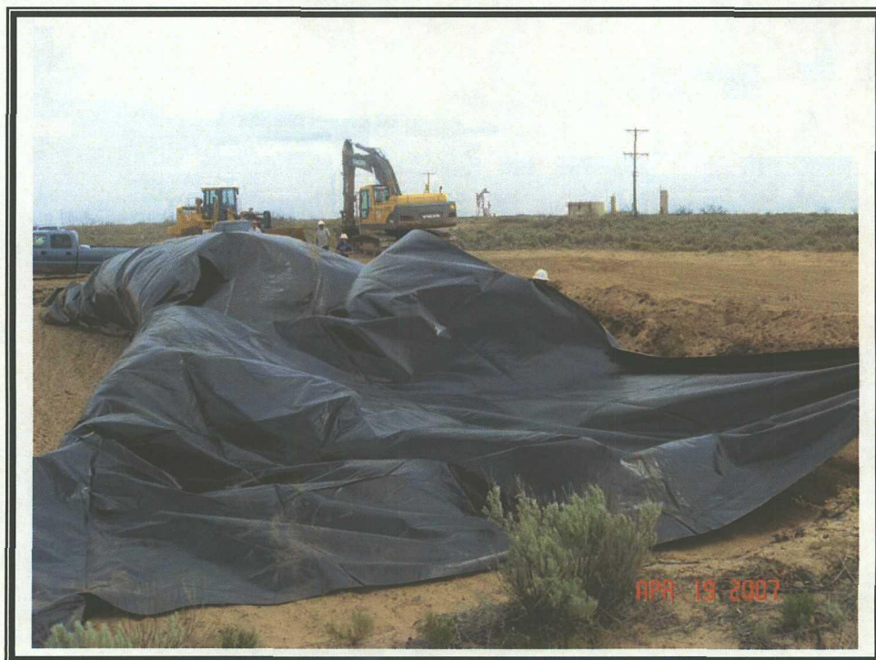
Installation of 20 mil Plastic Liner – MW-1 Area
