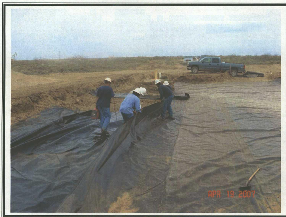
Installation of 20 mil Plastic Liner – MW-1 Area
