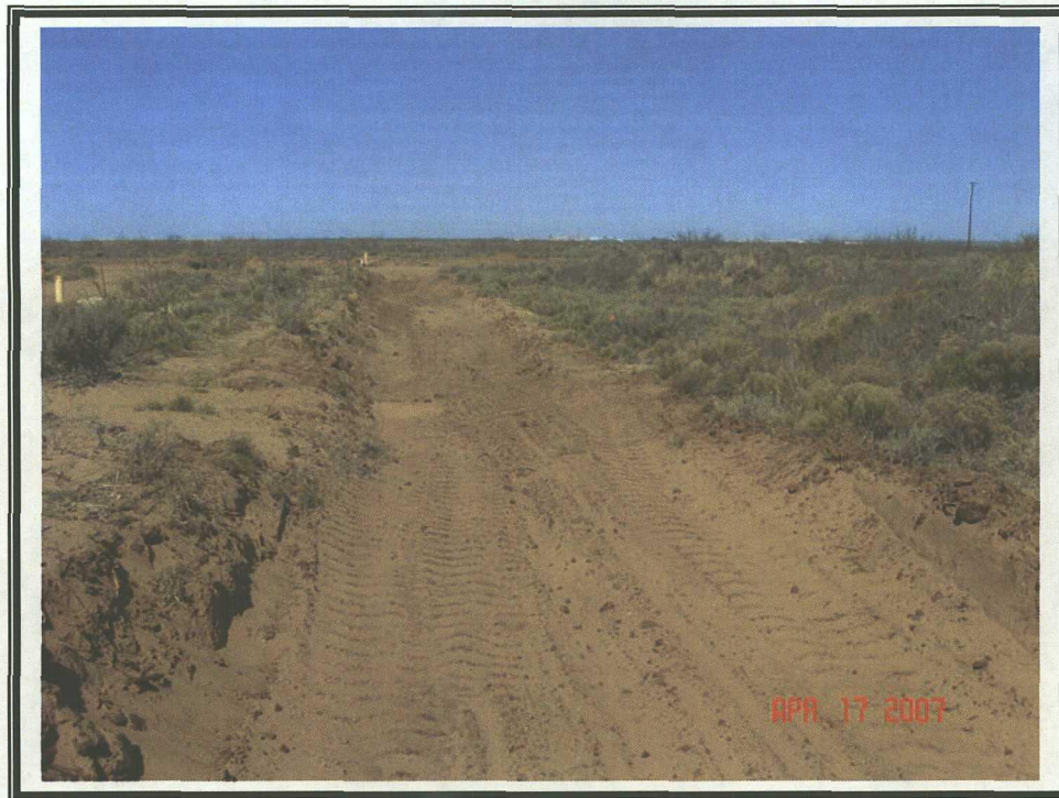
Excavation of Sluice Box
