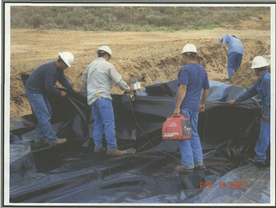
Installation of 20 mil Plastic Liner – MW-1 Area
