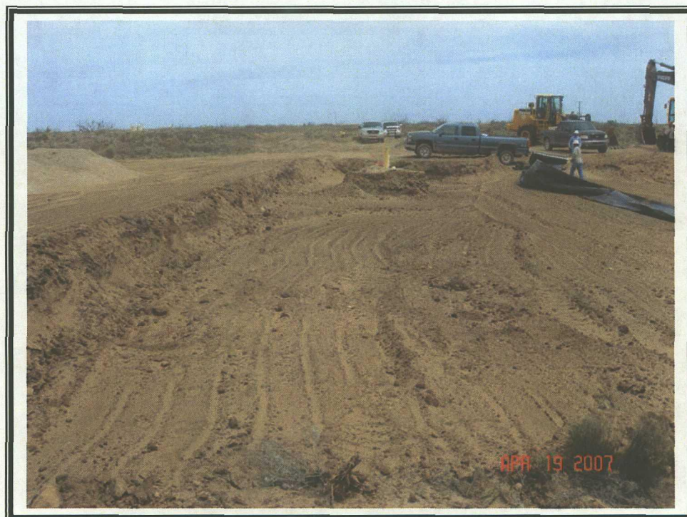
Installation of 20 mil Plastic Liner – MW-1 Area
