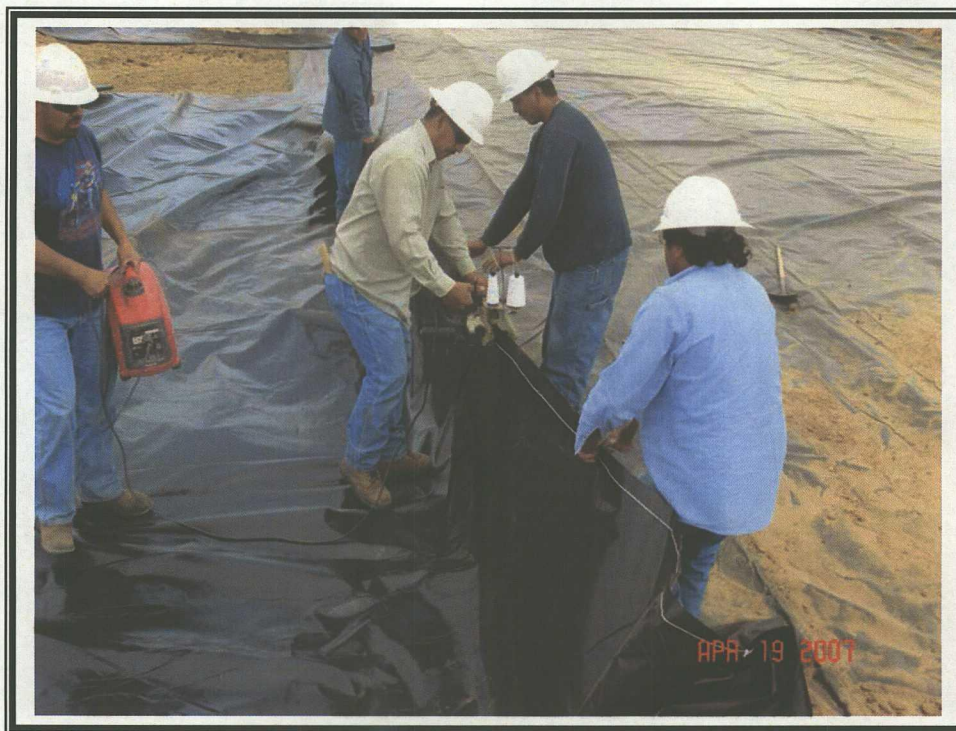
Installation of 20 mil Plastic Liner – MW-1 Area
