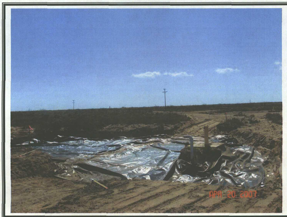
20 mil Plastic Lines – MW-2 Area
