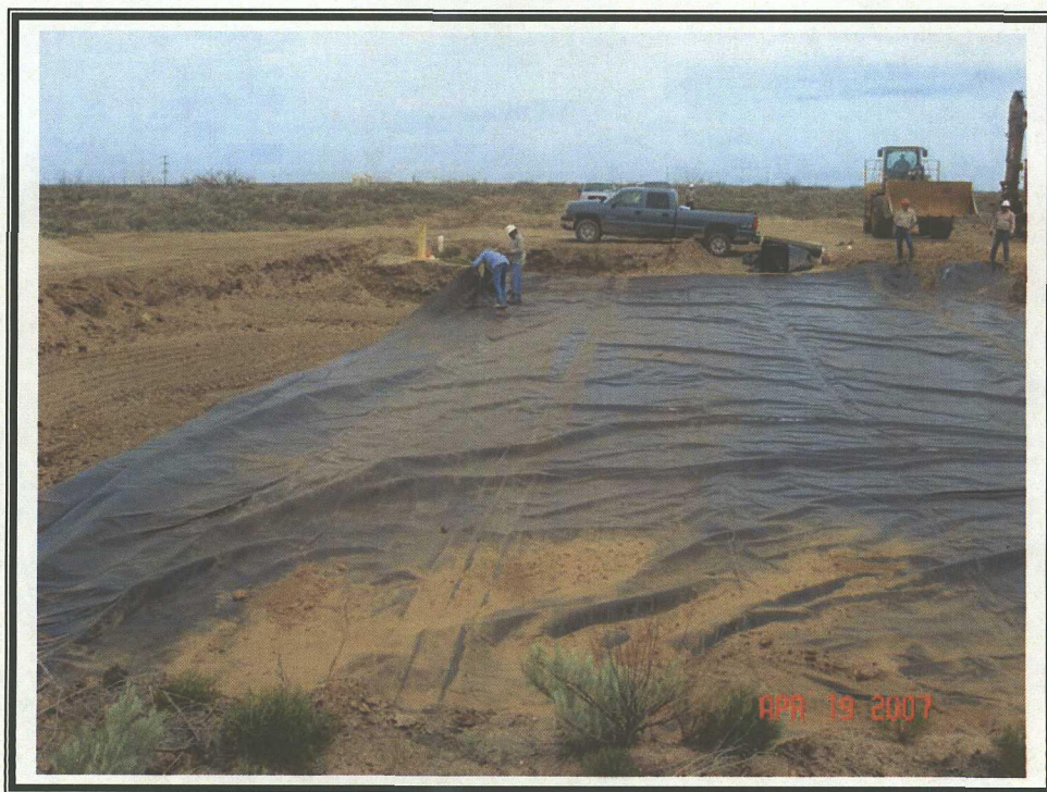
Installation of 20 mil Plastic Liner – MW-1 Area
