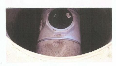
Figure 9: TK-6 325 Gallon Poly Waste Oil Tank in Fiberglass Vault
