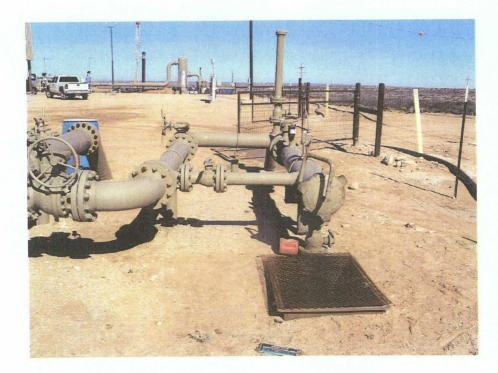
Figure 11: Pig Waste Steel Containment TK-8
