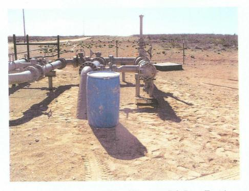
Figure 10: Pig Waste Steel Containment TK-7 and Temporary Poly Drum (Empty)
