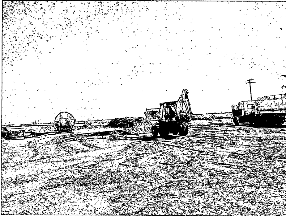
4/19/06 REMOVING IMPACTED CALICHE
