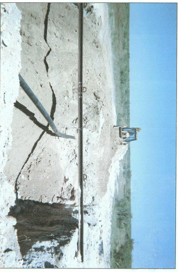
backfilling 30 x 30 x 12-ft-deep excavation
