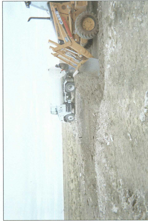
spreading imported topsoil on backfilled site
