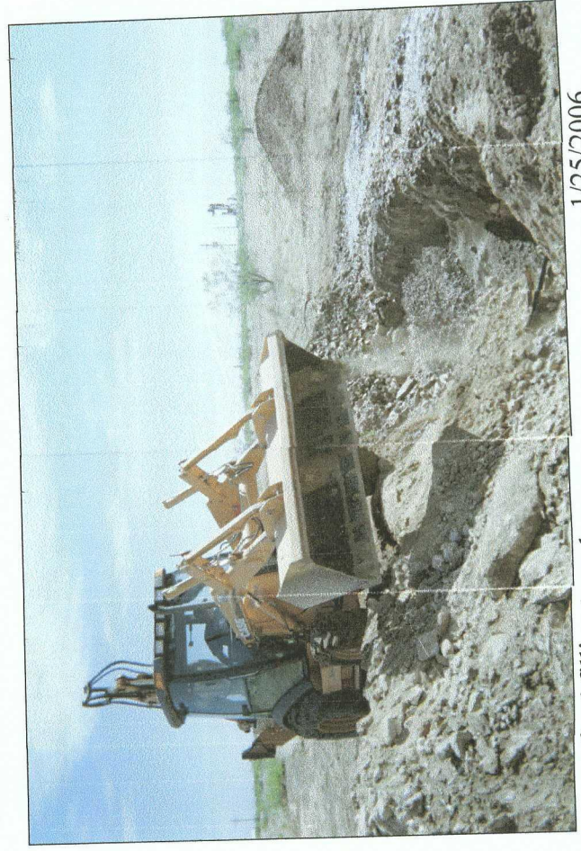
backfilling trench
