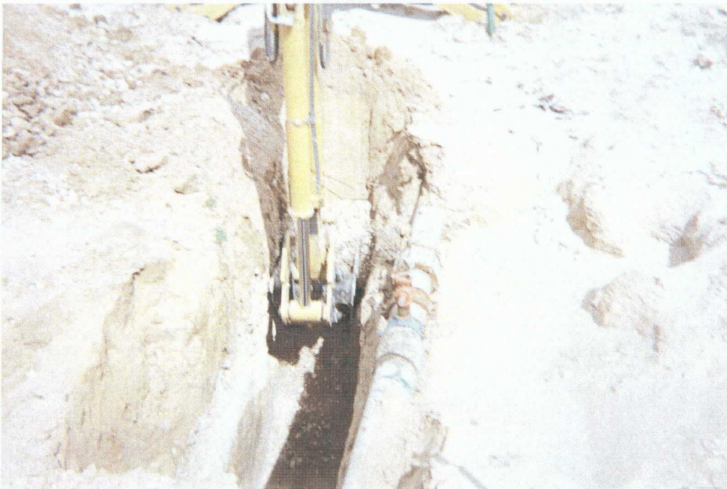
Photograph 2 – Soils evaluation at vent adjacent to former junction box.
