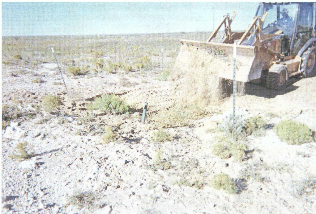
Photograph 3 – Backfilling of excavation.
