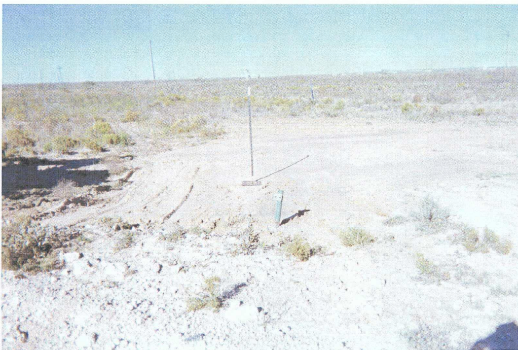
Photograph 4 – View of site following junction box removal. Note that a steel marker plat has been installed at the ground surface for future reference.
