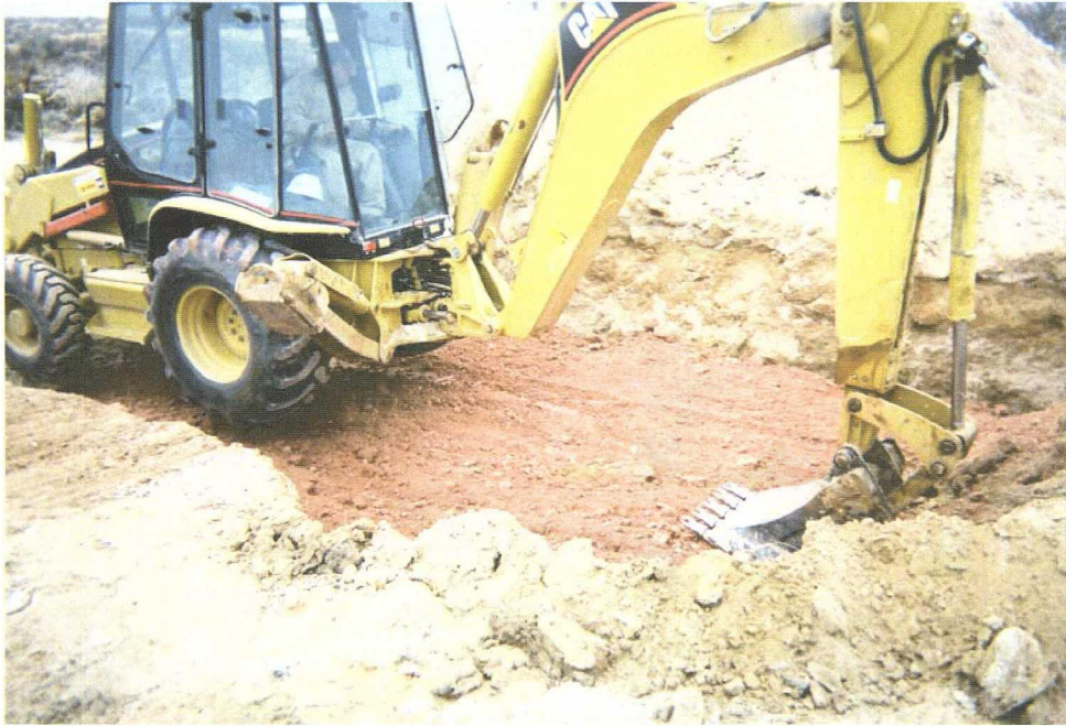
Figure 7: Compaction of clay layer
