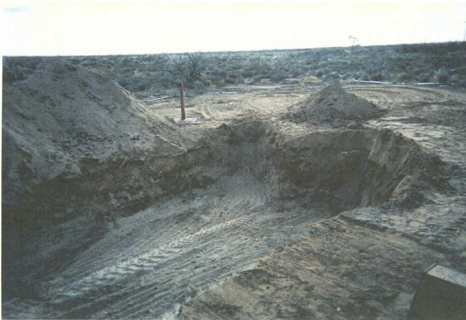
Figure 2: Excavation of site in preparation for ET Barrier, December 2006
