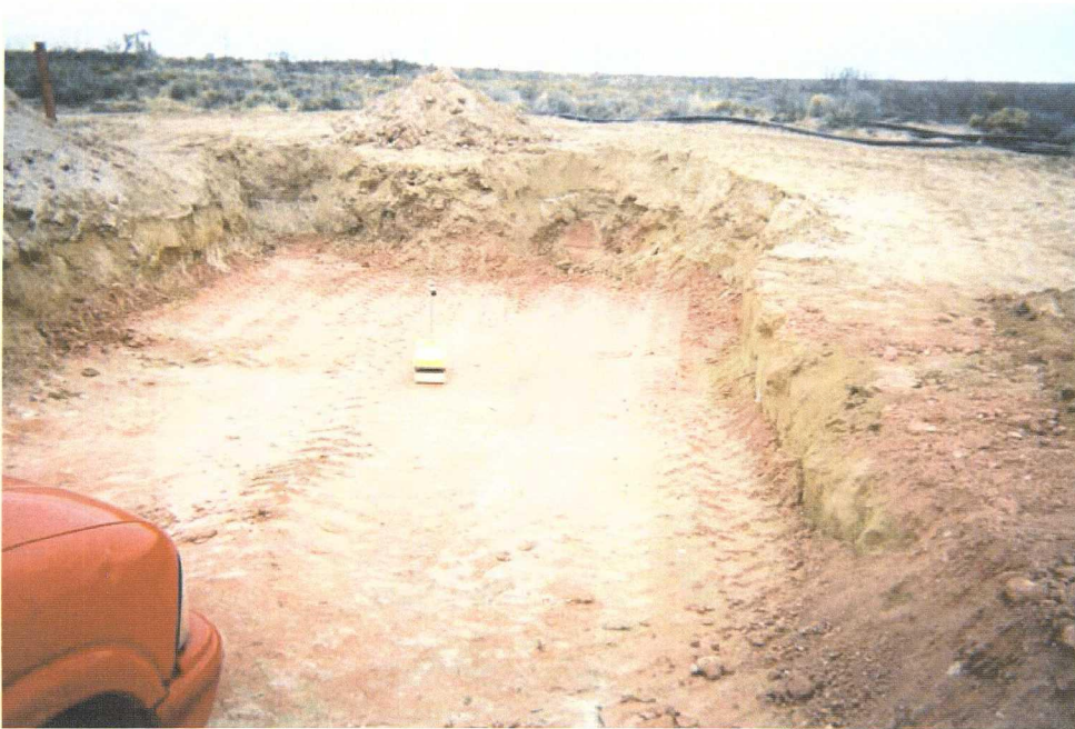
Figure 8: Density testing of clay lift
