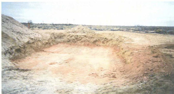
Figure 3. Installation of approved ET Barrier, December 2006.
