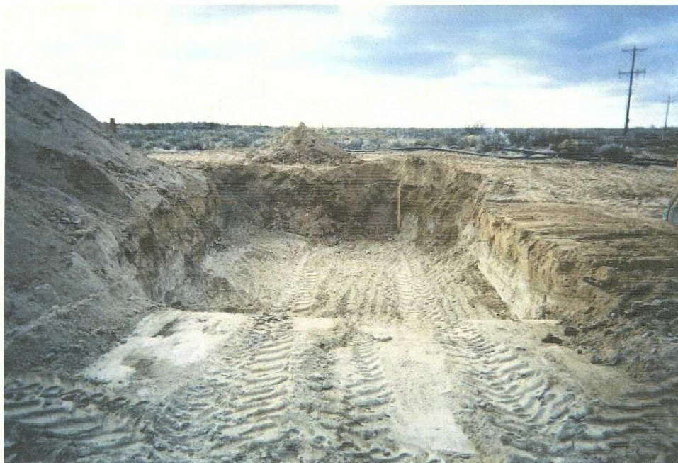
Figure 4: Preparation for installation of ET barrier
