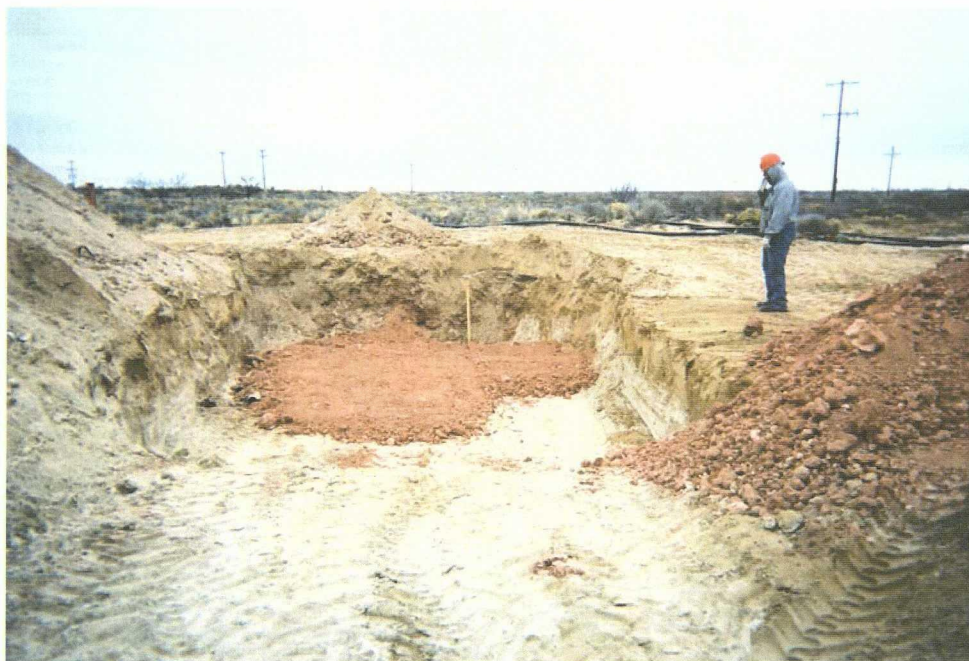
Figure 5: Placement of first clay lift on prepared surface
