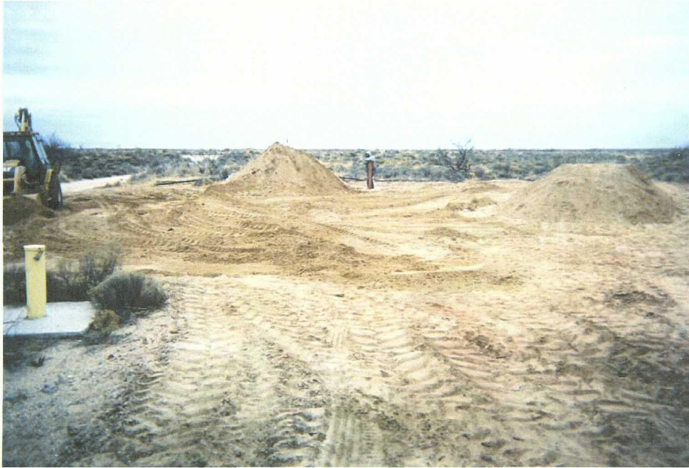
Figure 9: Placing topsoil over compacted clay
