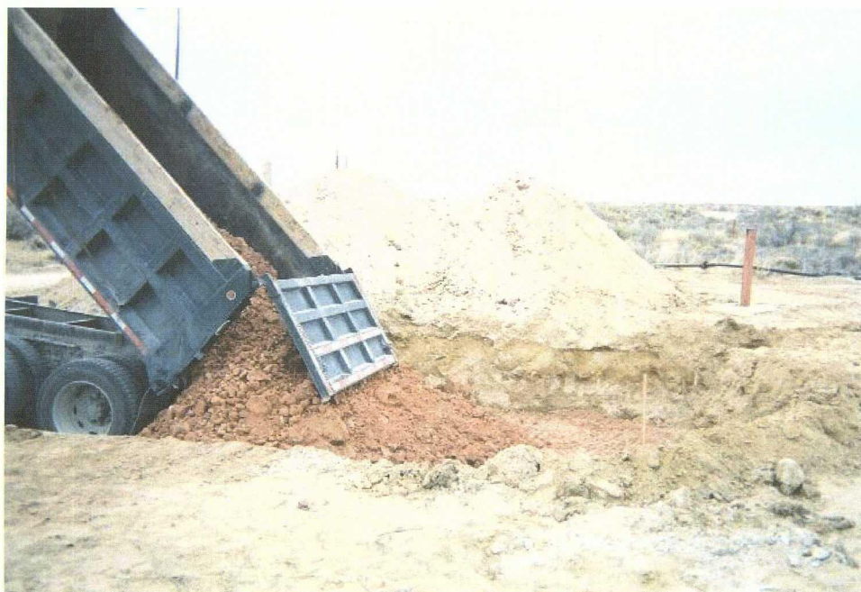
Figure 6: Delivery of clay for second lift
