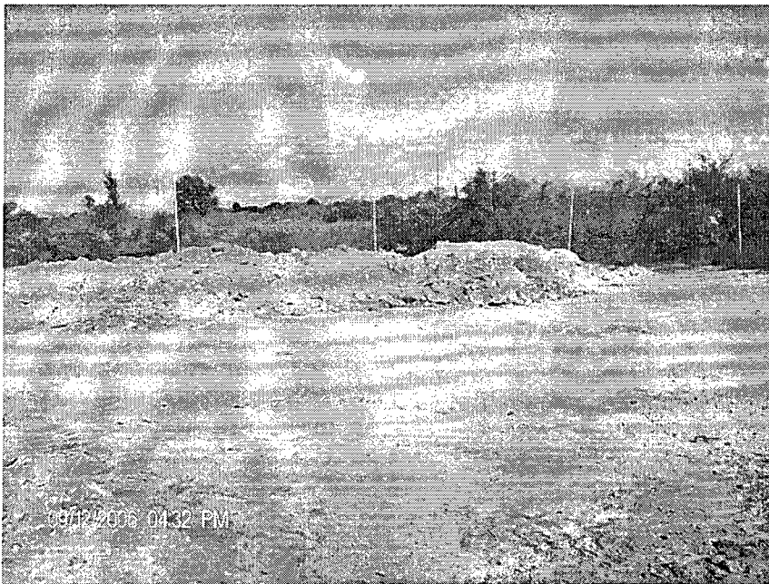
Figure 11: Segregated material for disposal
