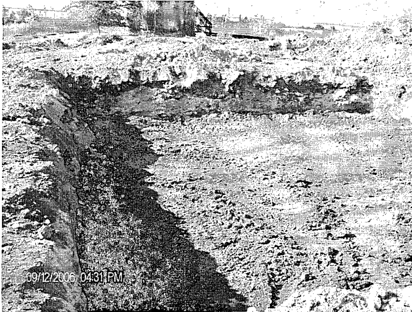
Figure 8: Clay placed in excavation
