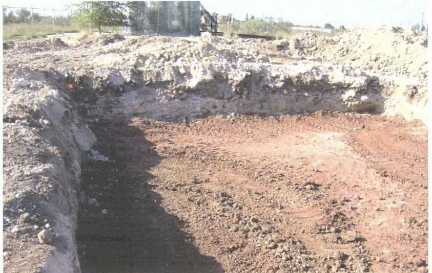
Figure 2. Clay barrier installed at four feet below ground surface at site.
