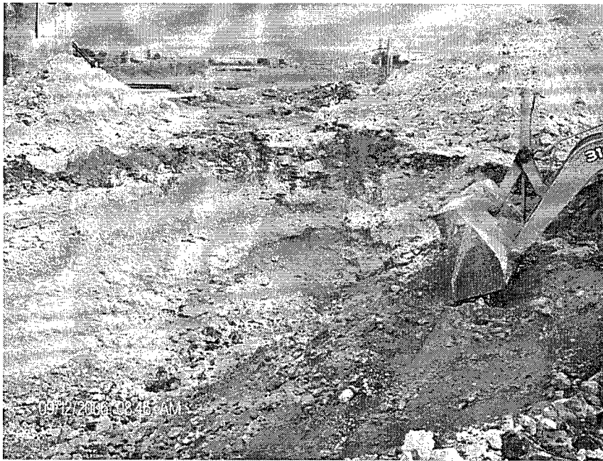
Figure 3: Backfilling excavation with blended soil
