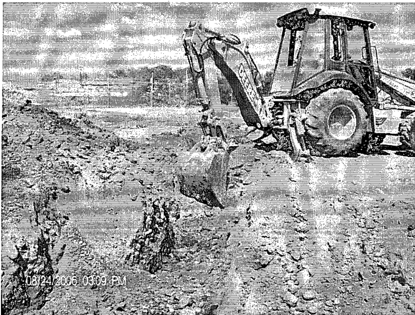
Figure 2: Digging out abandoned lines
