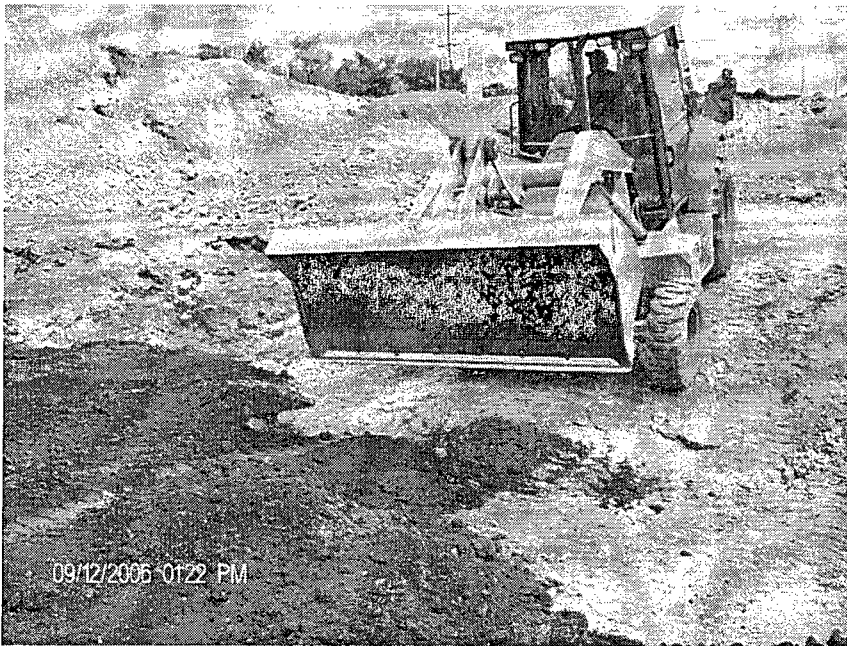
Figure 6: Compacting clay with equipment
