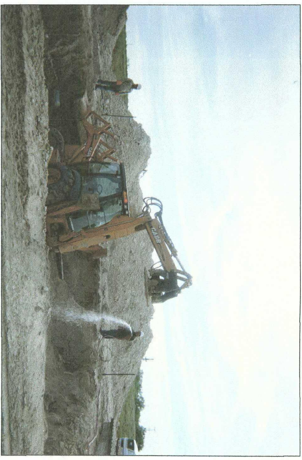
backfilling and compacting soil
