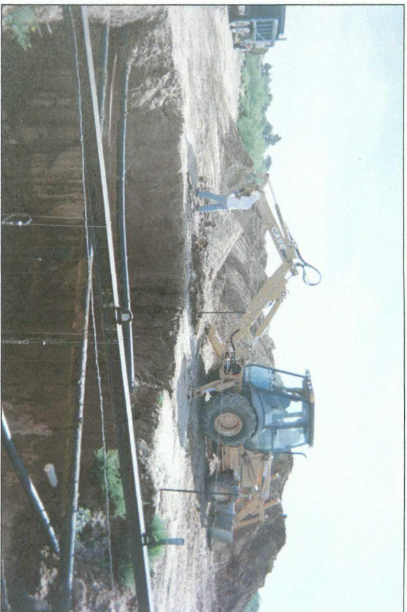
collecting soil samples from excavation
