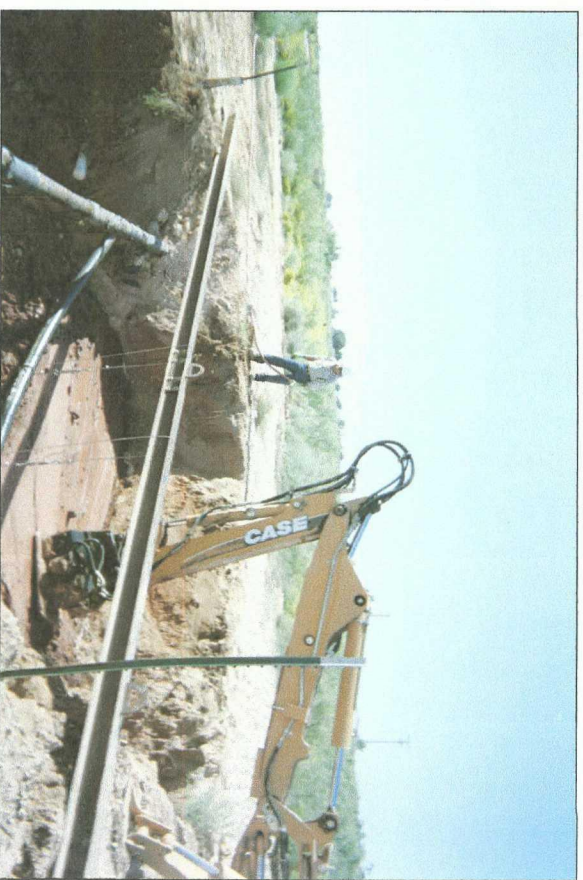
installing clay barrier at 6 ft BGS Sept. 2005
