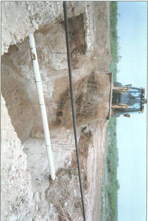
backfilling excavation
