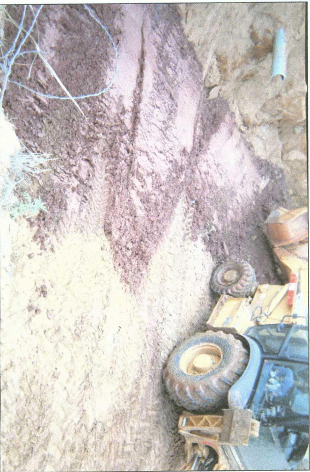
installing clay at 6 ft BGS
