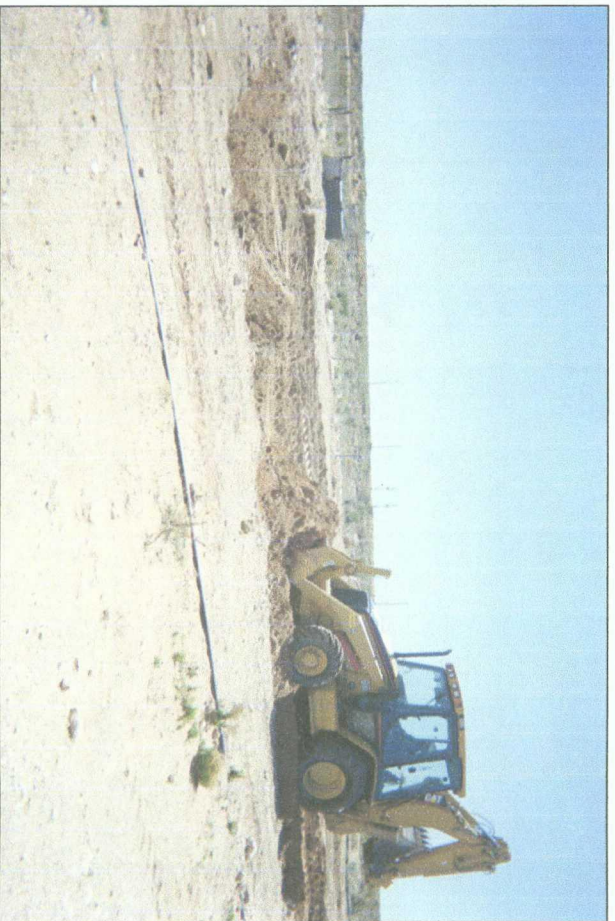
spreading imported soil and surface contouring
