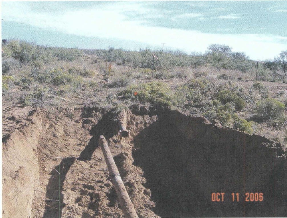
Photograph 1: Buried pipeline excavated, cut and capped with end clamp.
