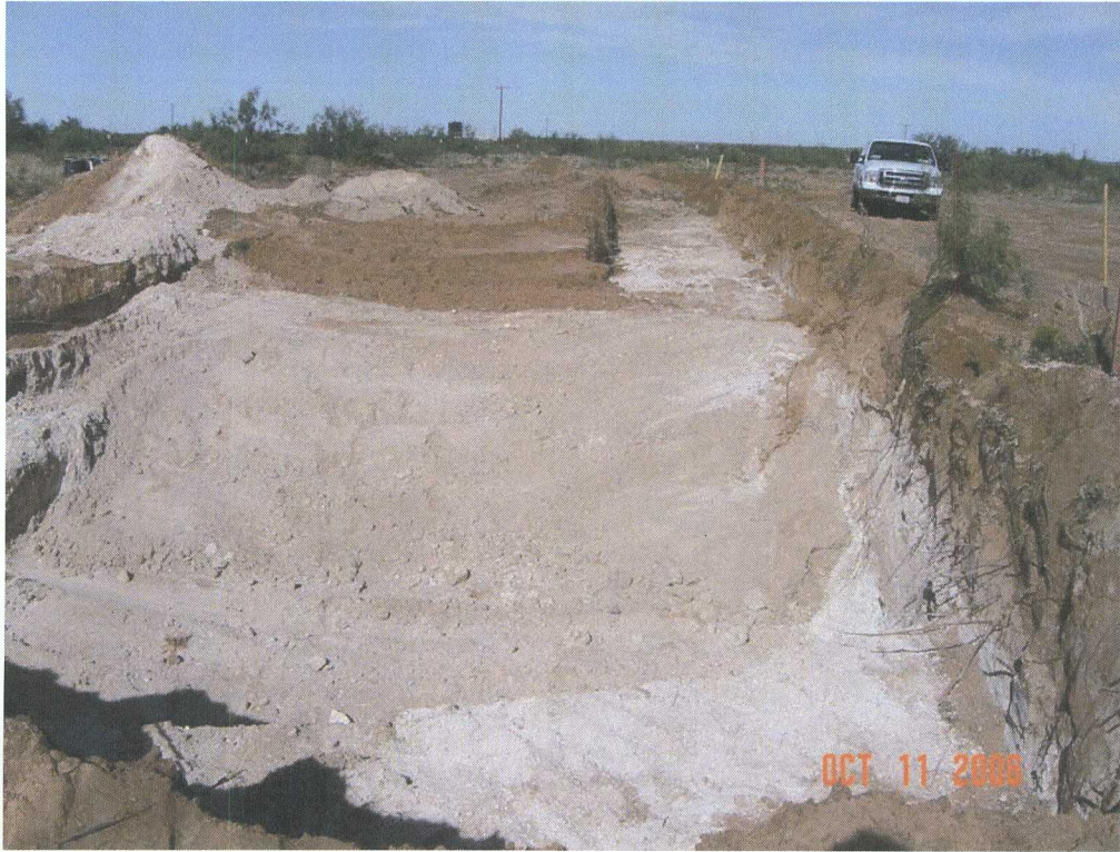
Photograph 3: Excavated area around monitor well MW-2.
