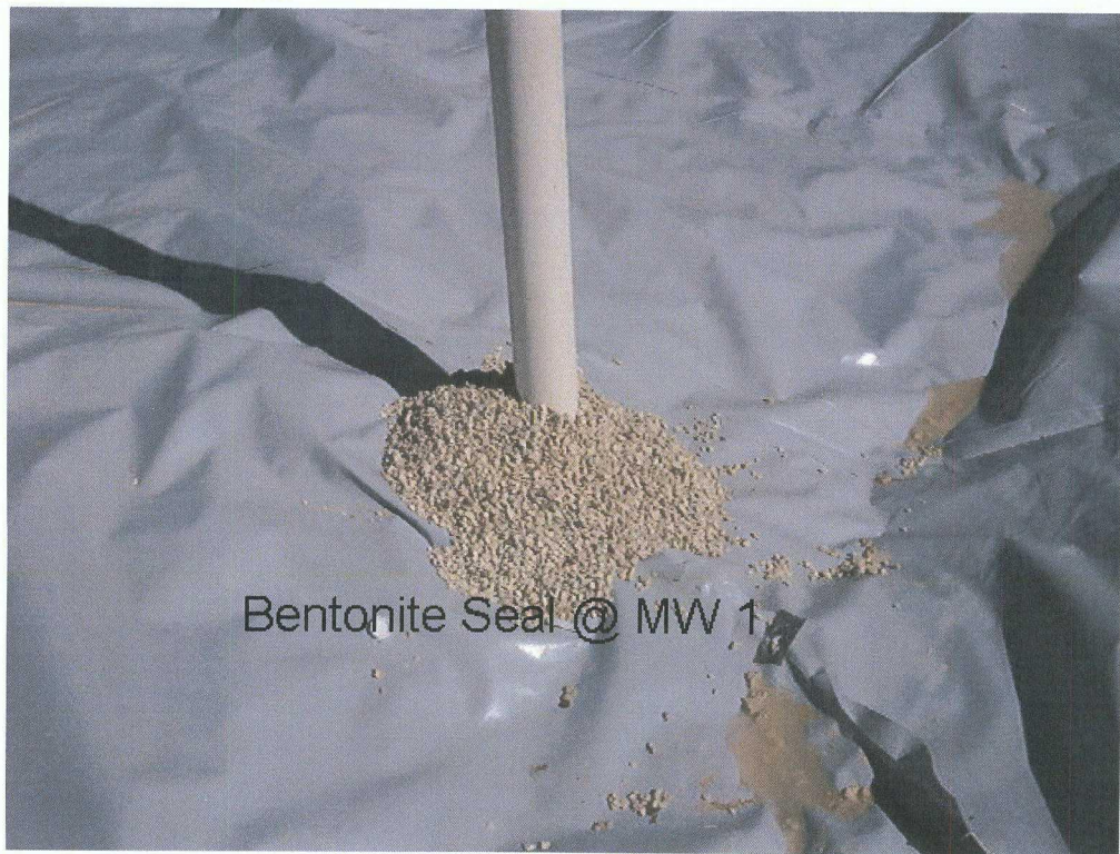
Photograph 10: Bentonite placed around monitor well to seal it in place.
