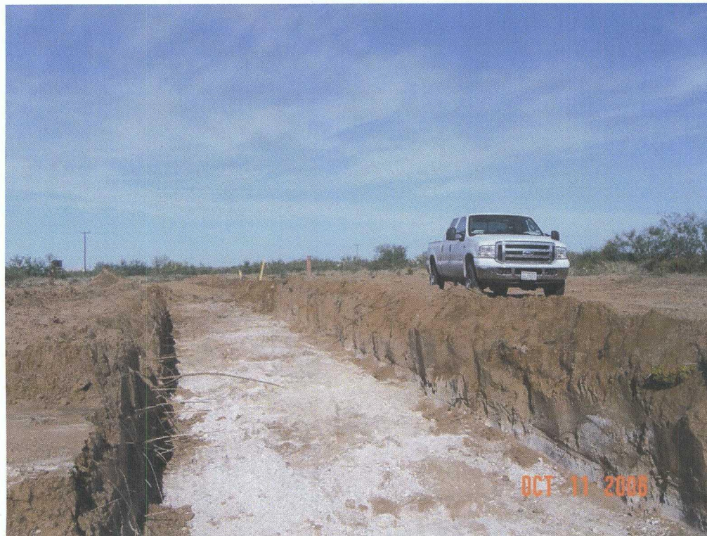
Photograph 2: 230 feet by 12 feet excavation of entire length of release (flow path).
