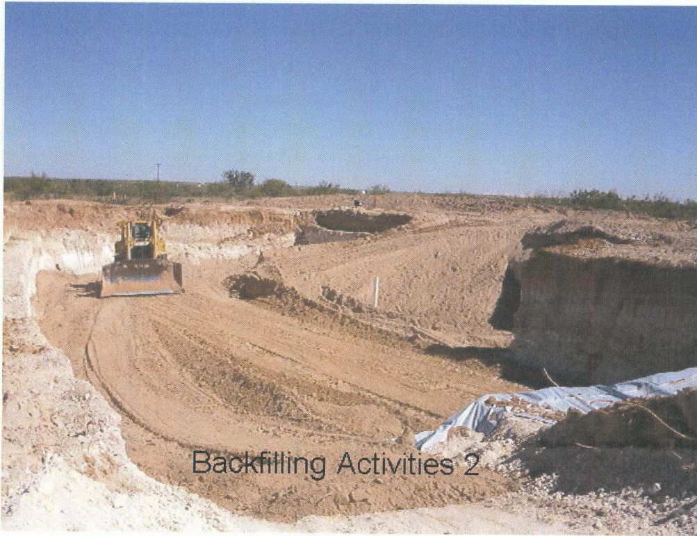
Photograph 11: Treated soil backfilled over liner.
