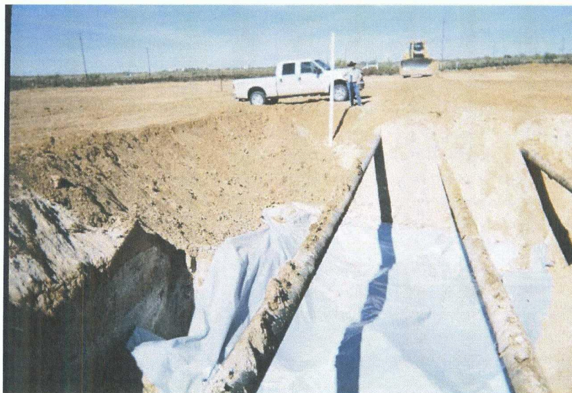
Photograph 8: Installation of upper liner with recovery well RW-1 in the background.
