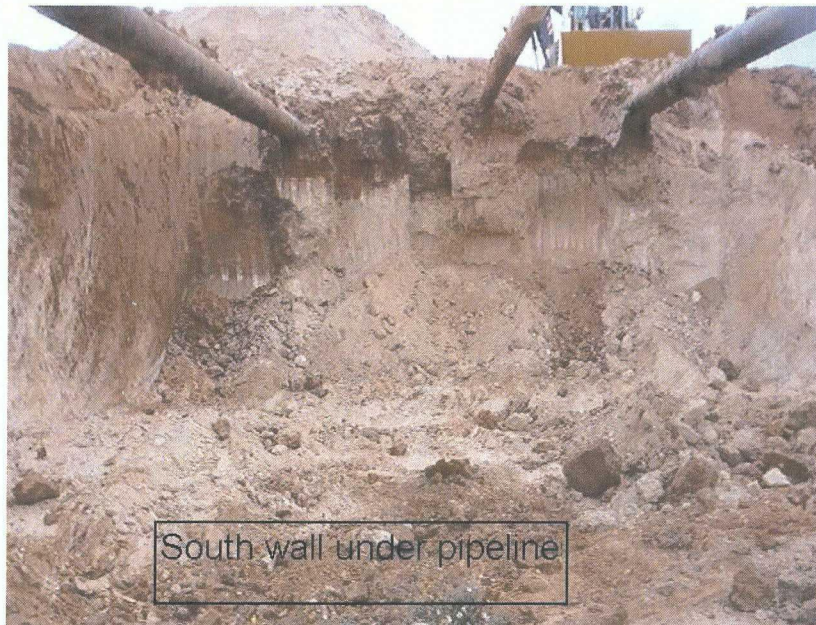
Photograph 7: View of the southernmost wall after over excavation activities.
