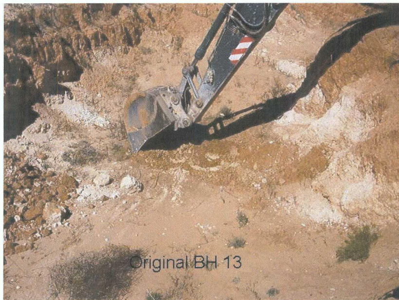
Photograph 6: Bottom hole sample BH-13 located in the northern portion of the excavation.
