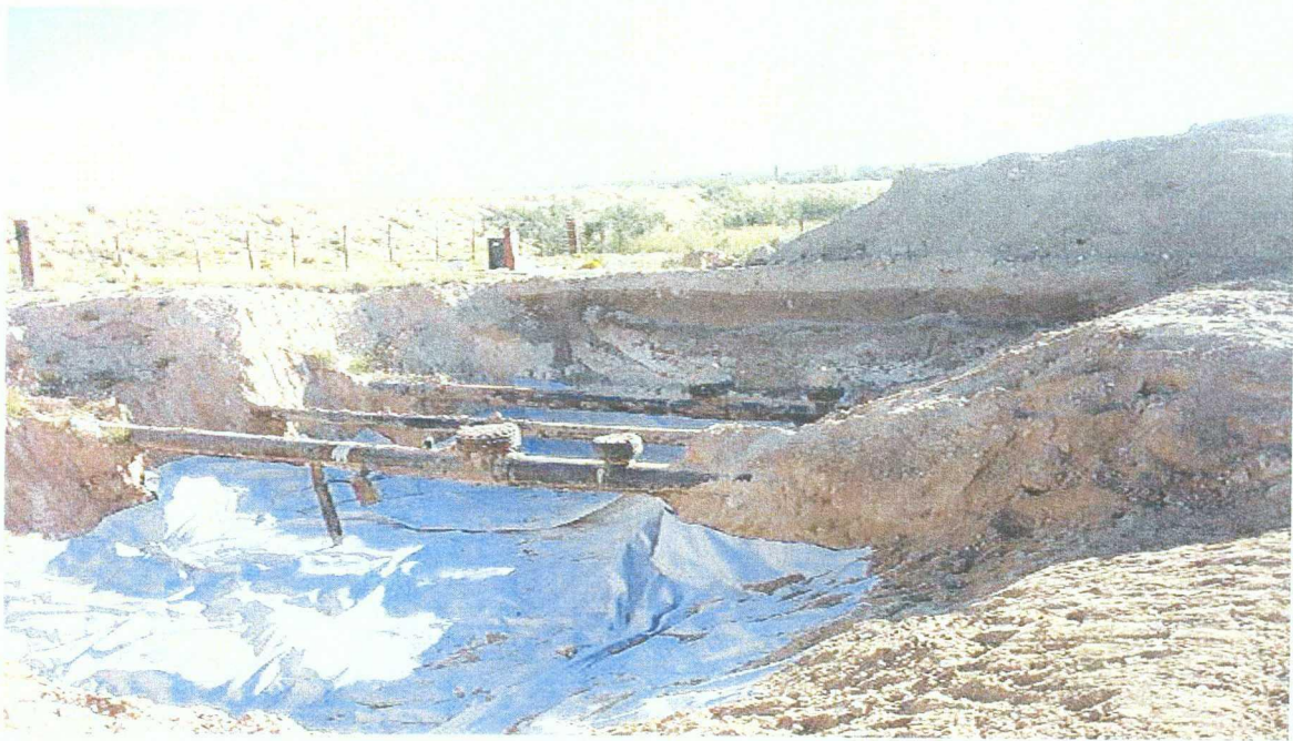
Photograph 2: Placement of 20-mil high-density polyurethane impermeable liner at the base of the excavation.
