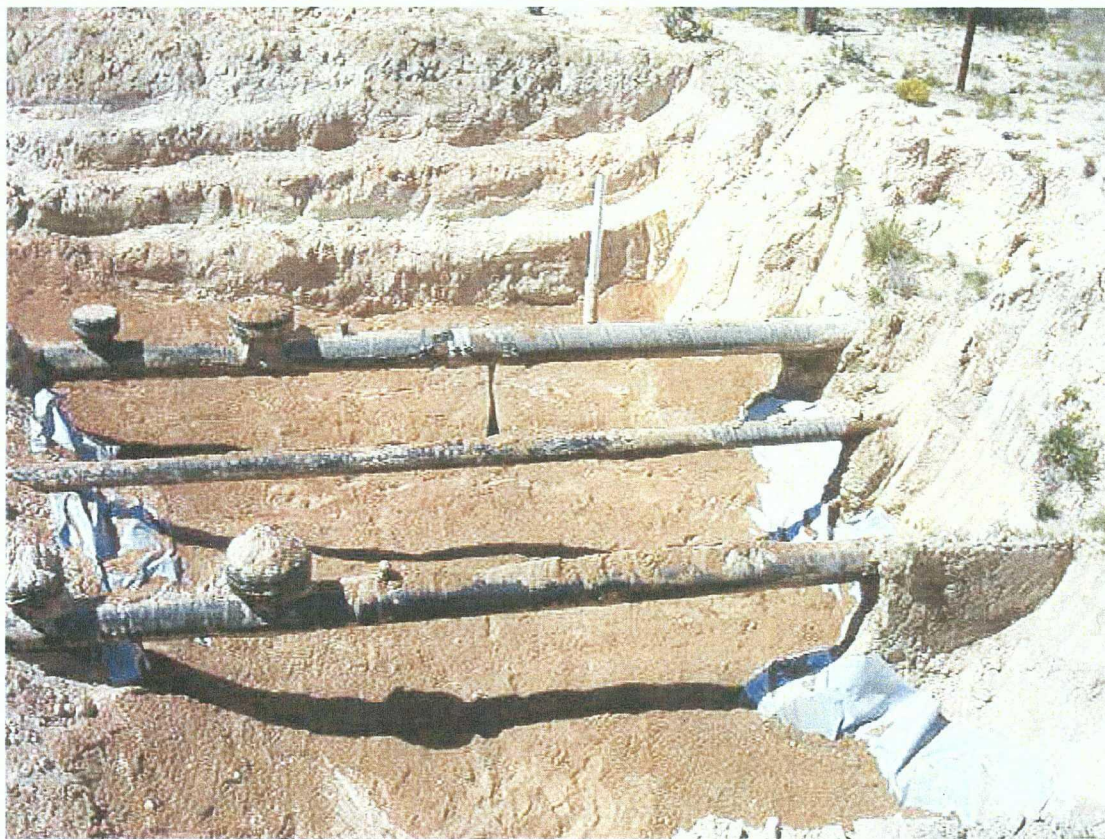
Photograph 3: Close-up view of the liner underneath the exposed pipeline.
