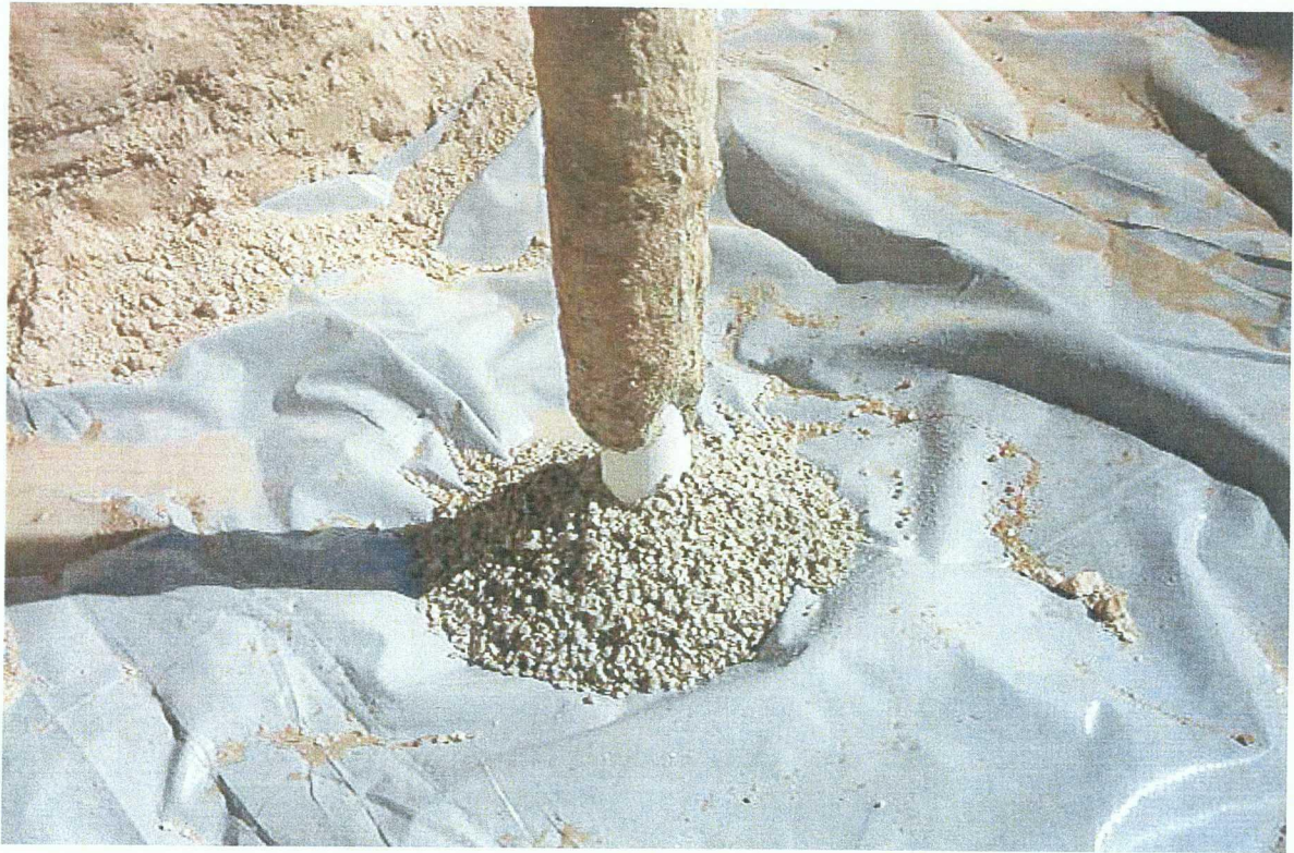
Photograph 5: View of the bentonite seal around the monitoring well MW-1.
