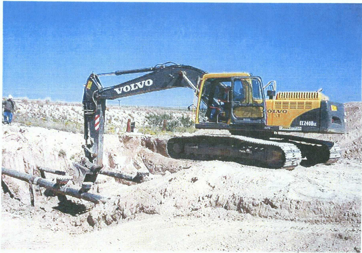
Photograph 1: View of the soil excavation underneath the exposed pipeline.
