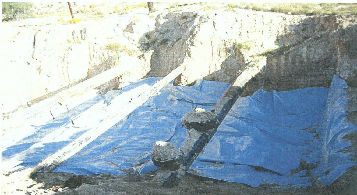
Photograph 3: Close-up view of the liner underneath the exposed pipeline.
