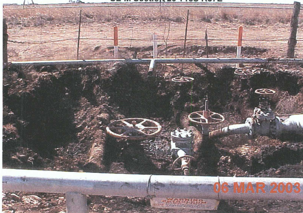
Photograph #3- Looking down on excavation at point of release.
