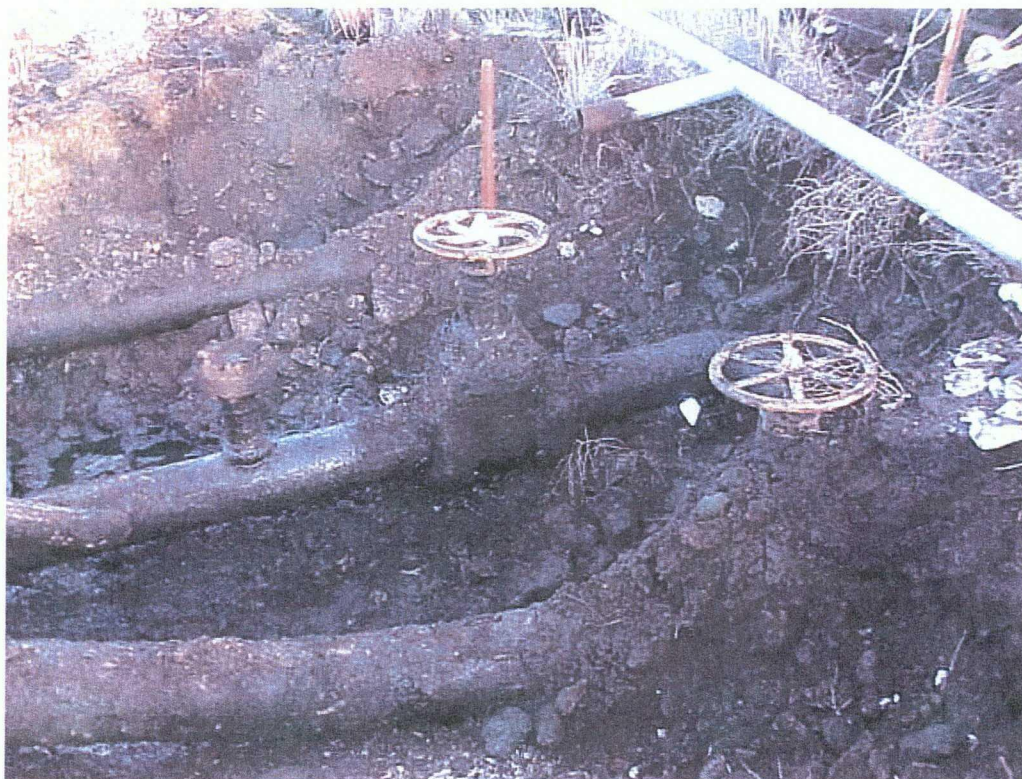
Photograph #4- Looking down on excavation at point of release.
