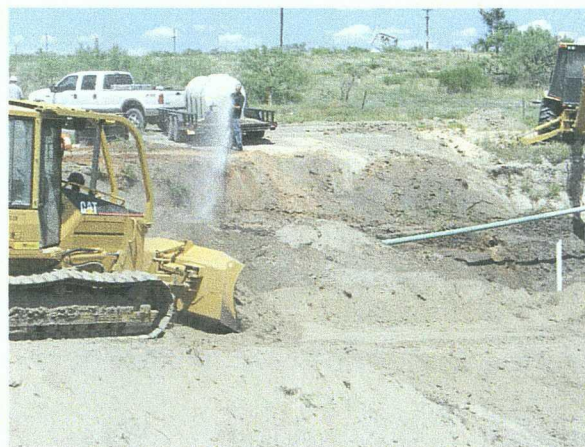
Photo #22 Hosing down the stockpiled material as it is being backfilled into the excavation.
