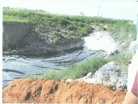
Photo #8 View to the southeast of the PVC liner on the floor of the excavation.
