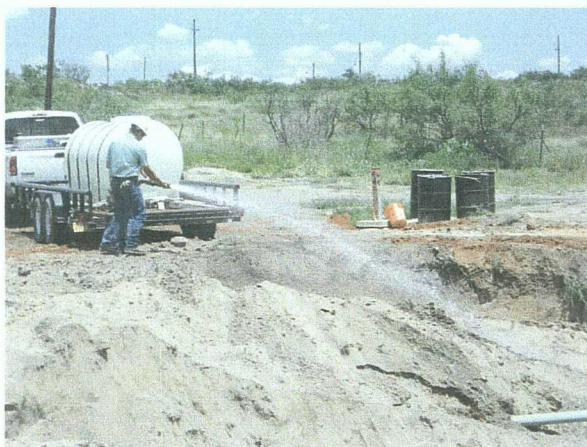
Photo #21 View to the northeast; hosing down the stockpiled material as it is being backfilled into the excavation.
