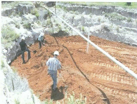
Photo #17 View to the east of sand being placed below the pipeline.
