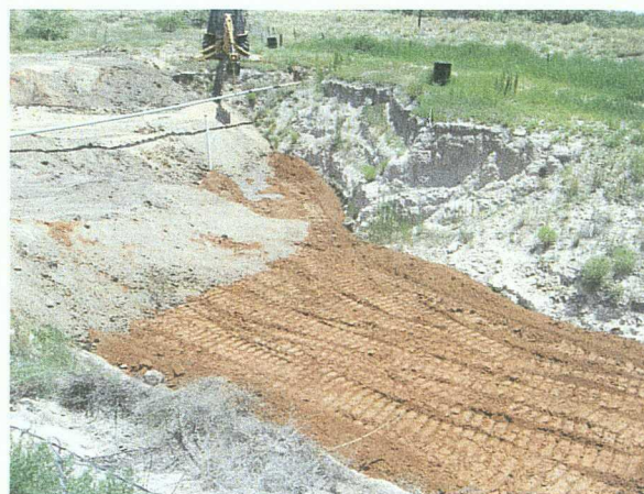
Photo #20 View to the northeast of stockpiled materials being placed over the sand at the excavation.
