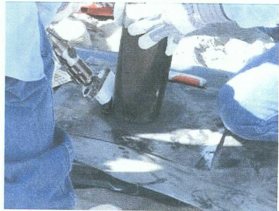
Photo #14 Sealing the monitor well TMW-1 in the floor of the excavation.
