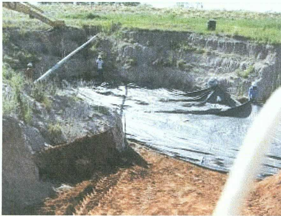
Photo #7 View to the northeast of the PVC liner being laid on the floor of the excavation.
