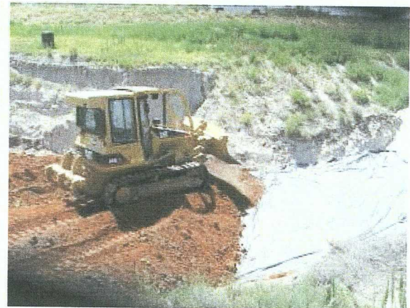
Photo #16 View to the east of sand being placed on the liner.
