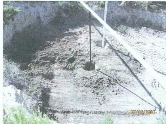
Photo #2 View of the floor of the excavation. Monitor well TMW-1 is visible in the back center of the photograph.
