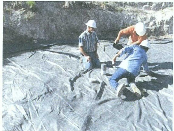
Photo #10 Laying the PVC liner on the floor of the excavation around monitor well TMW-1.
