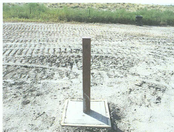
Photo #24 Monitor well TMW-1 completed with steel riser and concrete pad.
