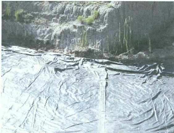
Photo #9 Central portion of the excavation with the PVC liner on the excavation floor.
