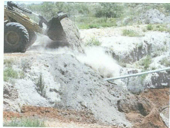
Photo #18 Begin backfilling the stockpiled material at the site.
