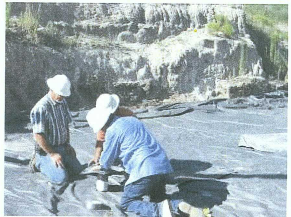
Photo #12 Sealing monitor well TMW-1 at the base of the excavation.
