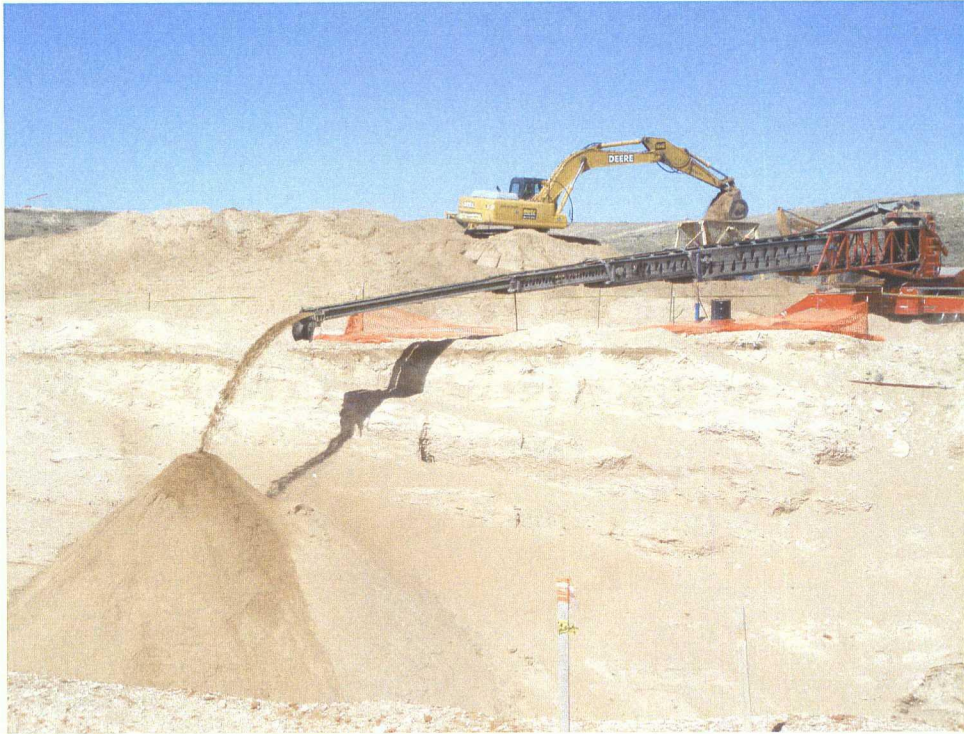
Photograph 7. Backfilling activities at the North Site using the tele-belt, view looking northwest. Photograph taken February 27, 2007.
