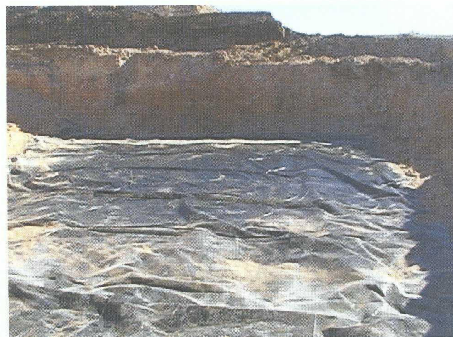
DT-27 – Liner Installed
