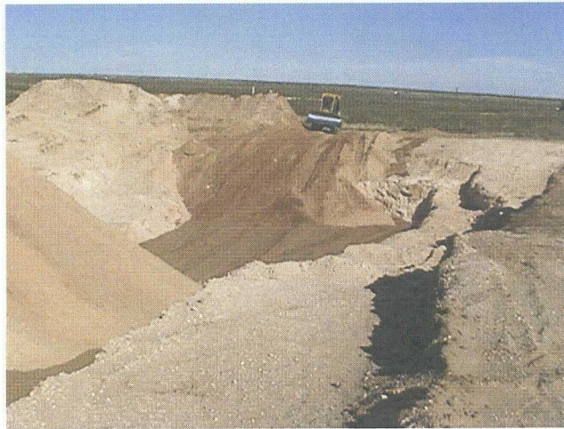
DT-27 – Backfill Over Liner
