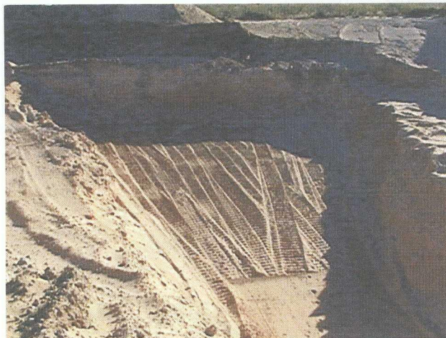
DT-27 – Prepared for Liner Installation
