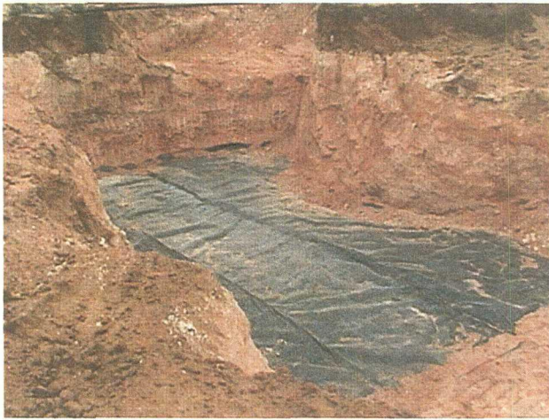
JALMAT 22A – Liner Installed
