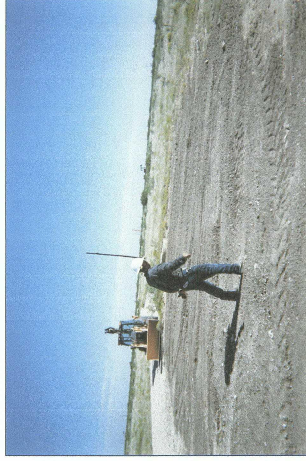
seeding backfilled surface
