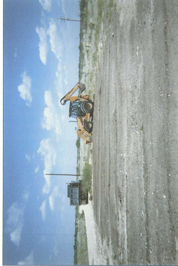
spreading clean, imported soil on surface
