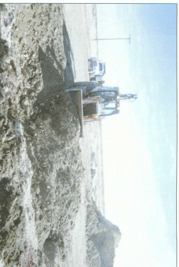
backfilling excavation
