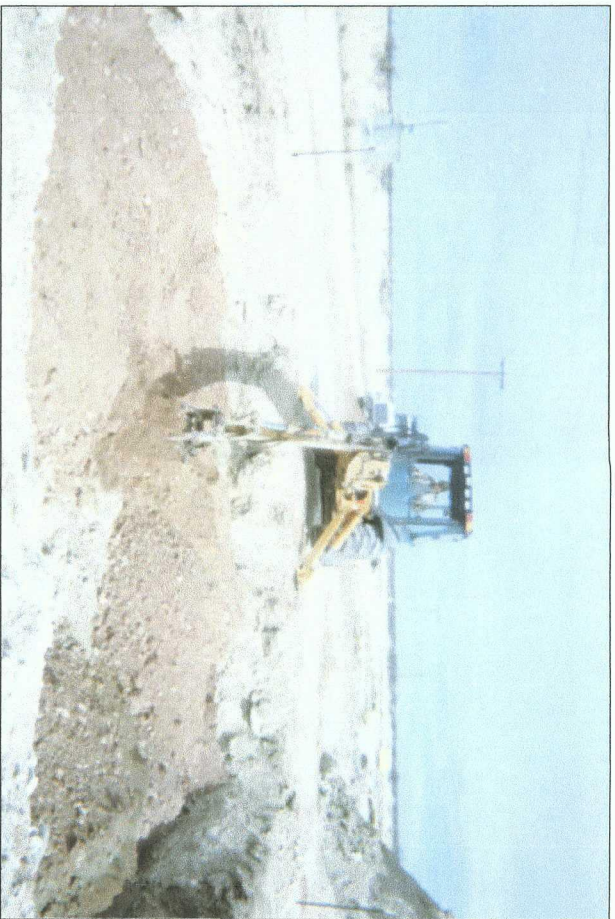
installing clay barrier at 6 ft
