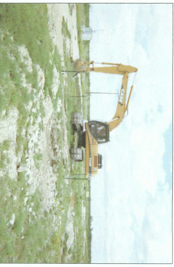
preparing for initial trackhoe delineation trench
