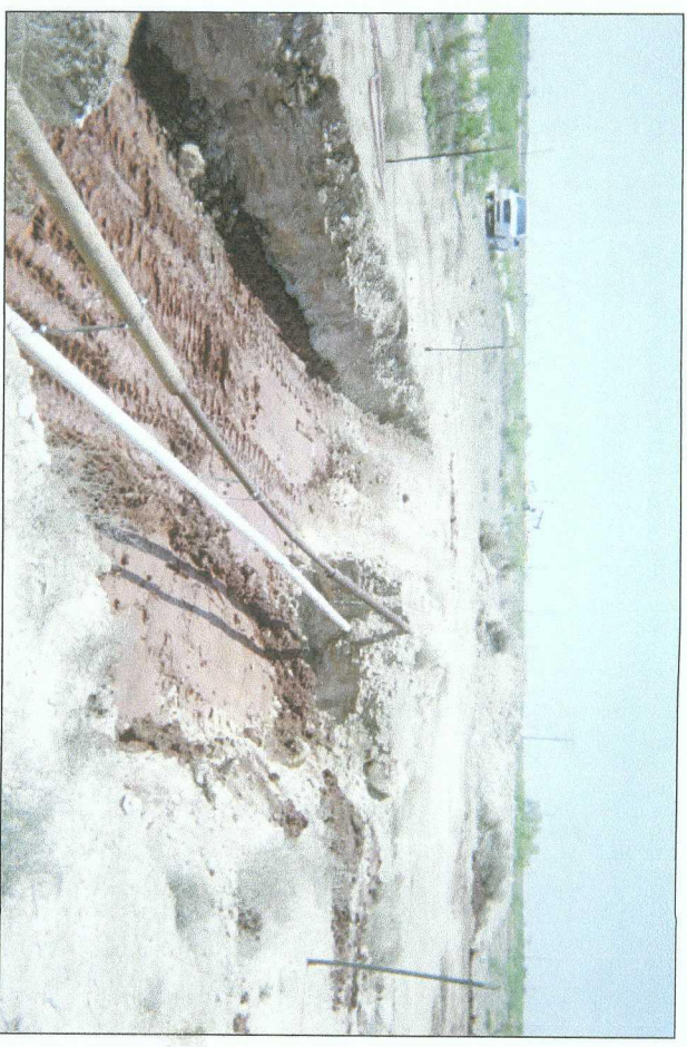
clay barrier at 6 ft BGS
