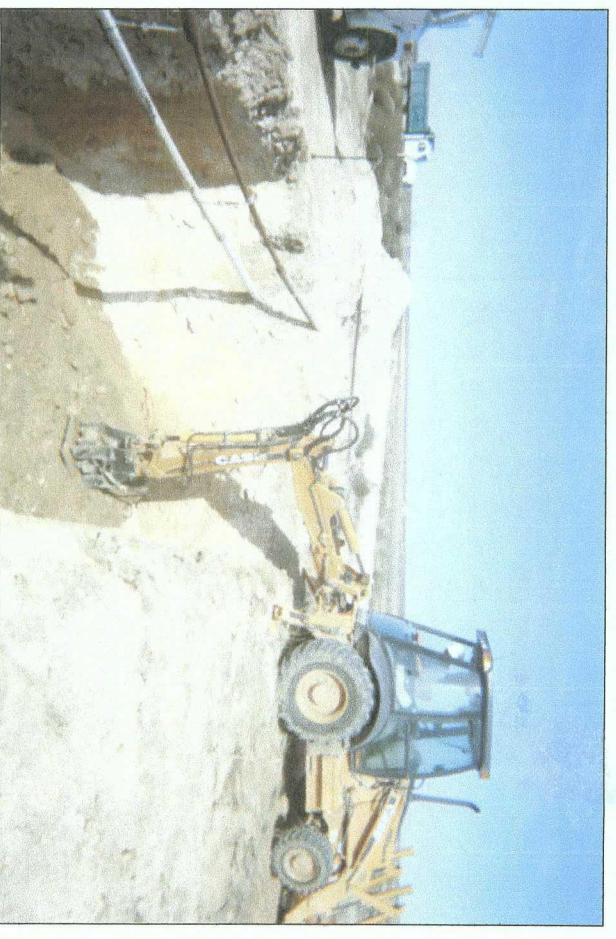
compacting backfill
