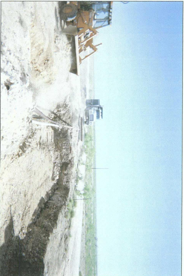
backfilling on top of clay
