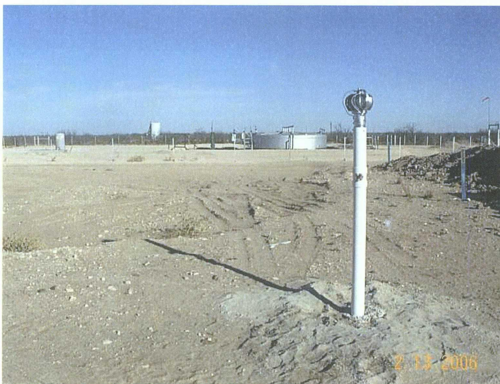
View facing east showing passive vapor extraction well at location of boring B-1.
