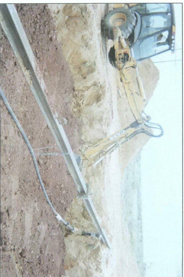
installing clay barrier at 6 ft
