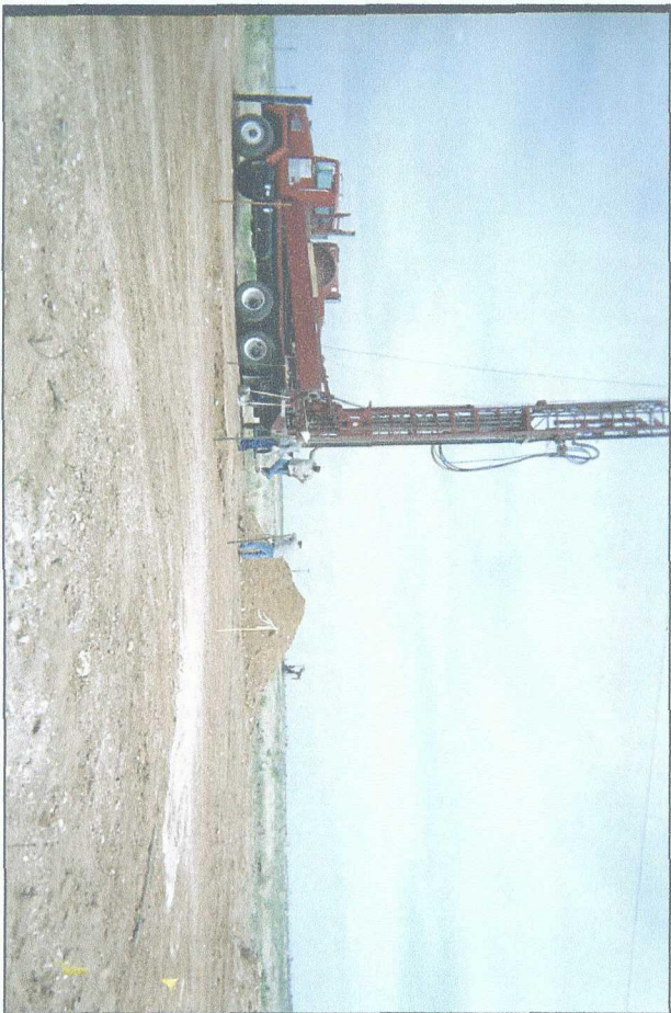
delineation soil borings at backfilled site
