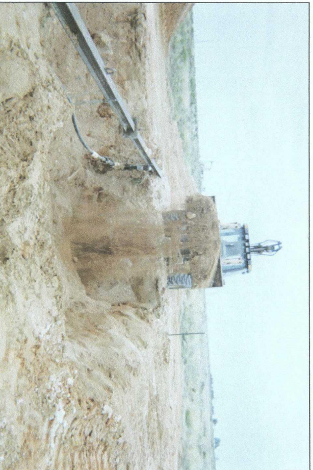
backfilling final 30 x 30 x 12 ft excavation
