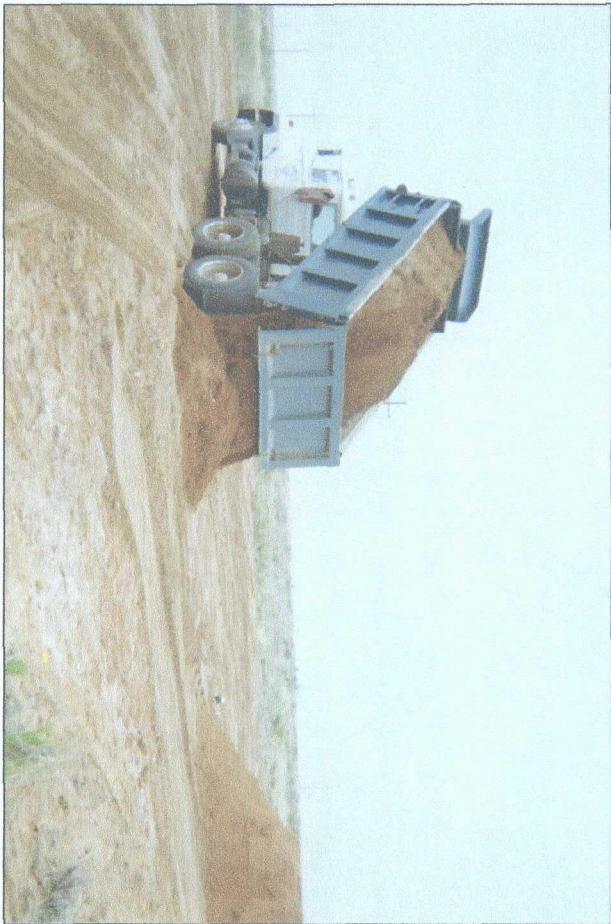
delivering topsoil to backfilled site
