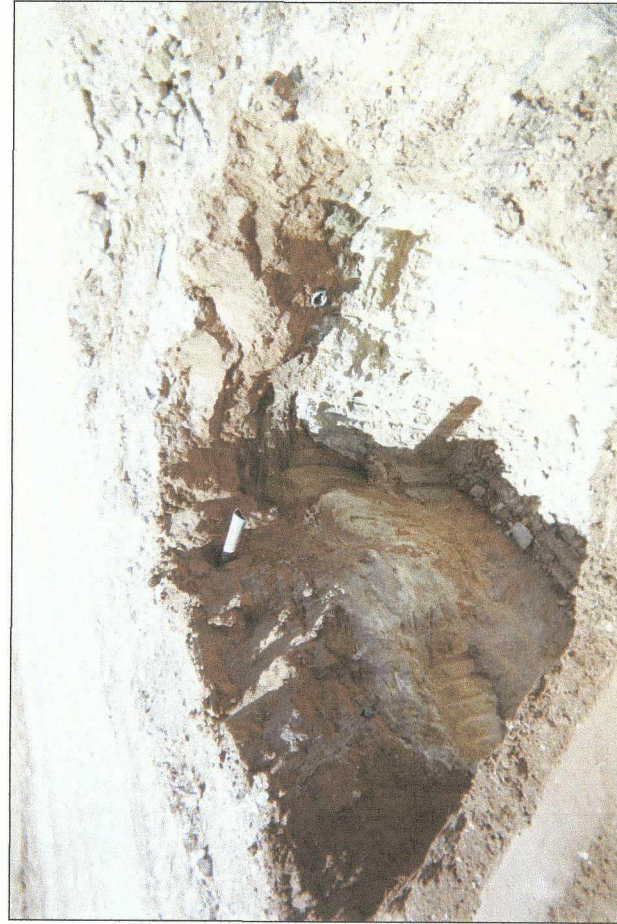
final 8 x 6 x 4-ft excavation at former box site
