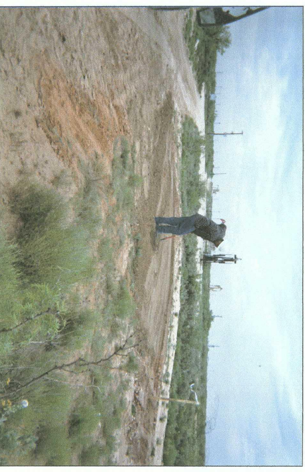
seeding imported topsoil of backfilled site
