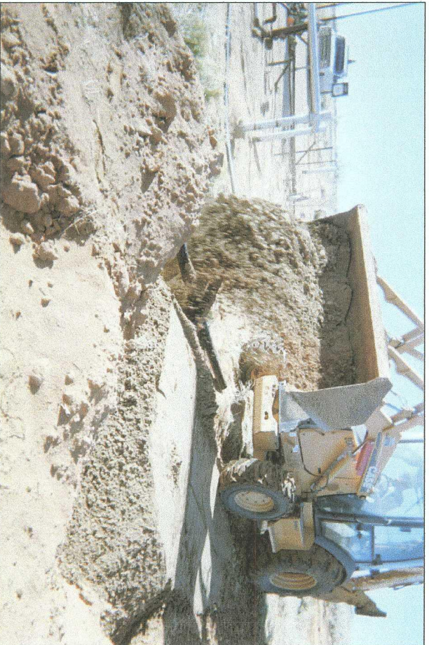
backfilling with imported soil
