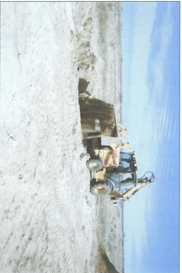
backfilling 10 x 10 x 12-ft excavation
