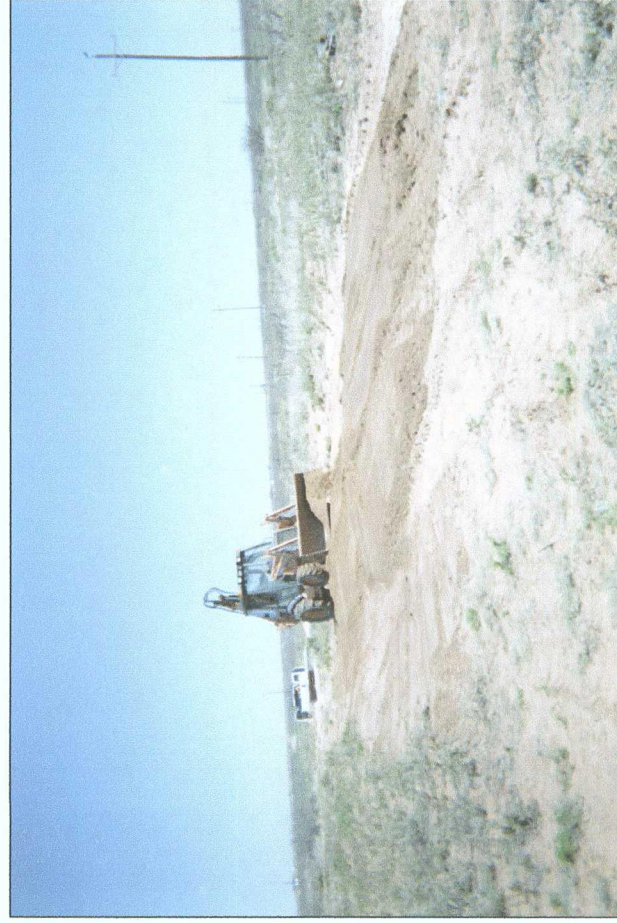
backfilling site with clean, imported soil
