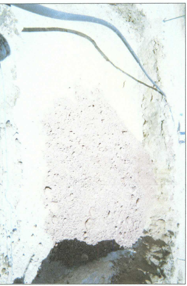
clay in excavation backfilled to 6 ft; ready for barrier installation
