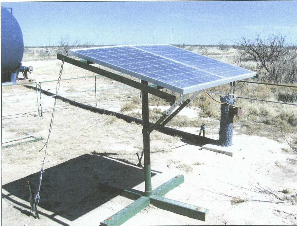
Figure 6- Solar powered groundwater recovery 1 system at Rice Vacuum SWD N-6-1 location.
