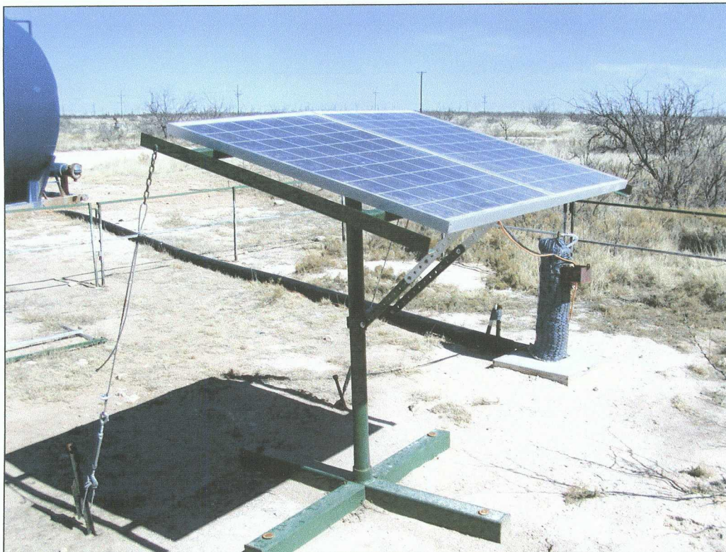
Figure 6- Solar powered groundwater recovery 1 system at Rice Vacuum SWD N-6-1 location.
