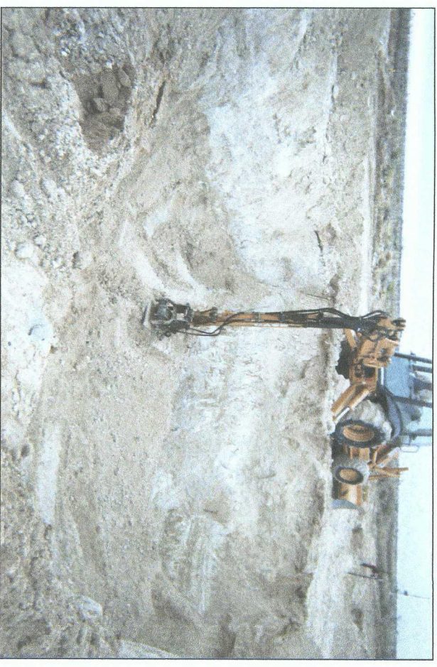
compacting backfill in 25 x 20 x 12 ft excavation 1/29/2007
