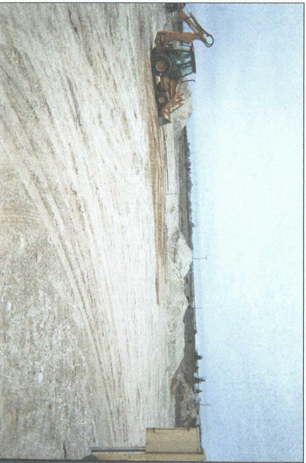
spreading clean, imported soil on top of backfilled site 1/30/2007
