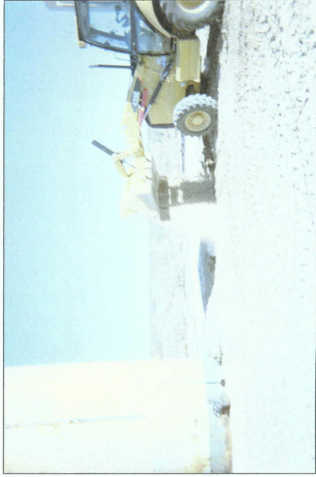
backfilling trench and repairing battery pad
