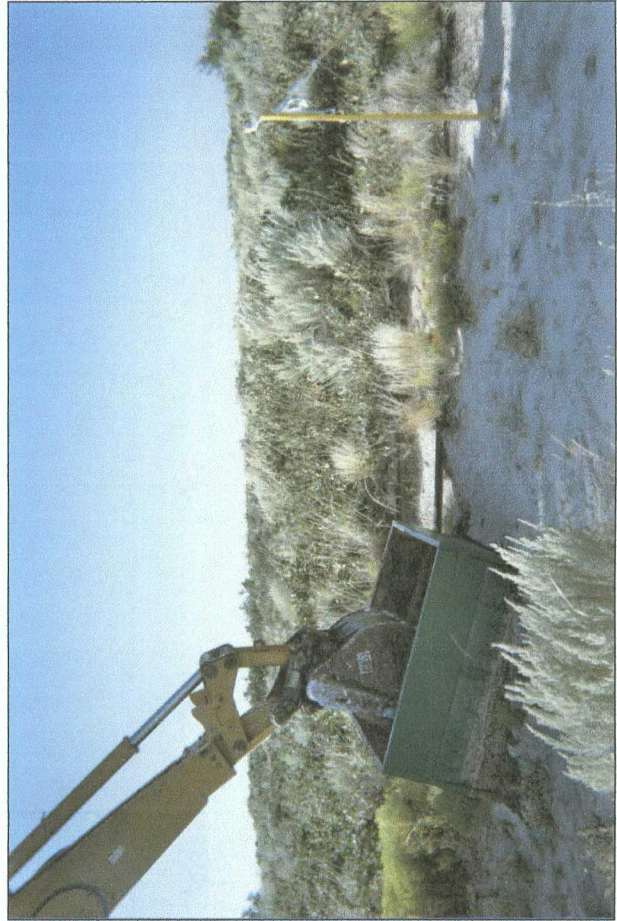
removing old junction box (junction eliminated)
