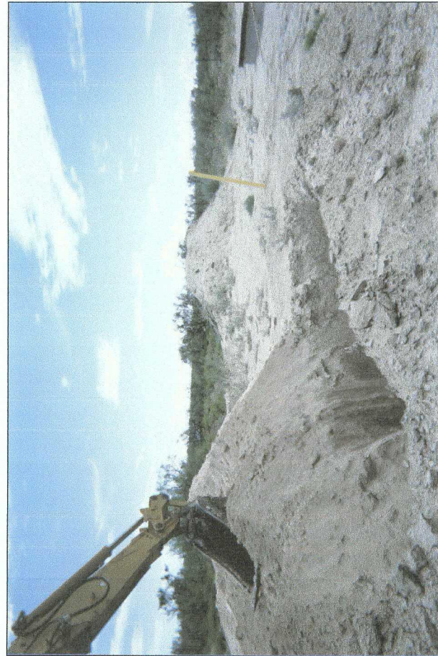
backfilling trench
