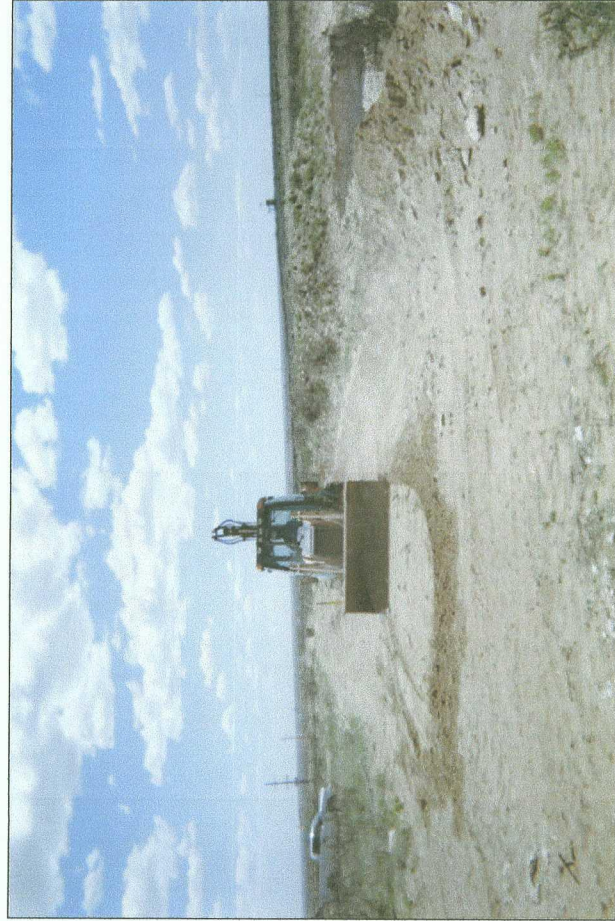
spreading clean, imported soil over backfilled site
