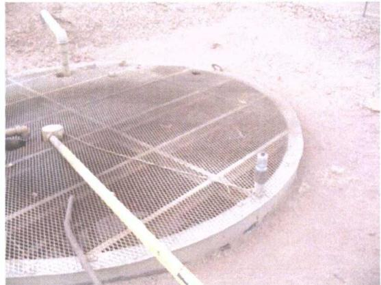
**Photo 5:** Cap for leak detection system has been installed.
