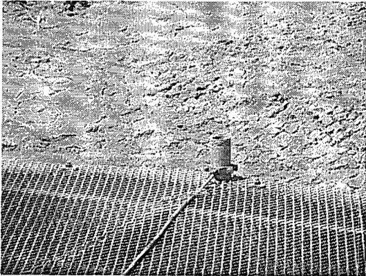
Photo 6: Leak detection lid is missing on BGT.
