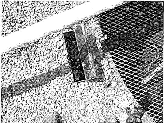
Photo 3: BGT leak detection system is full of fluids.
