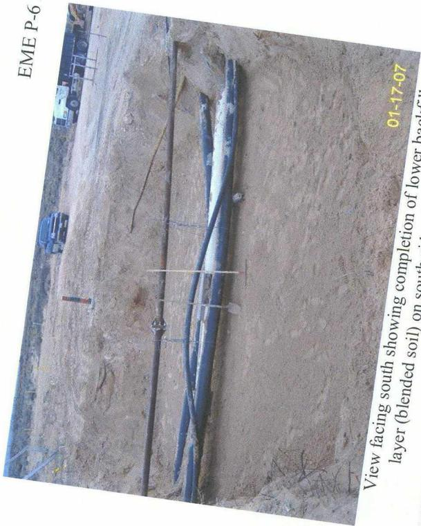
View facing south showing completion of lower backfill layer (blended soil) on south side of excavation.
