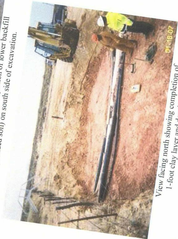
View facing north showing completion of 1-foot clay layer and density testing.
