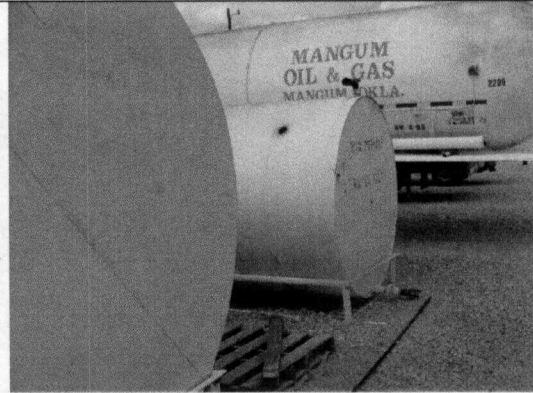
Photo 9: Saddle tanks within eroded bermed area.
