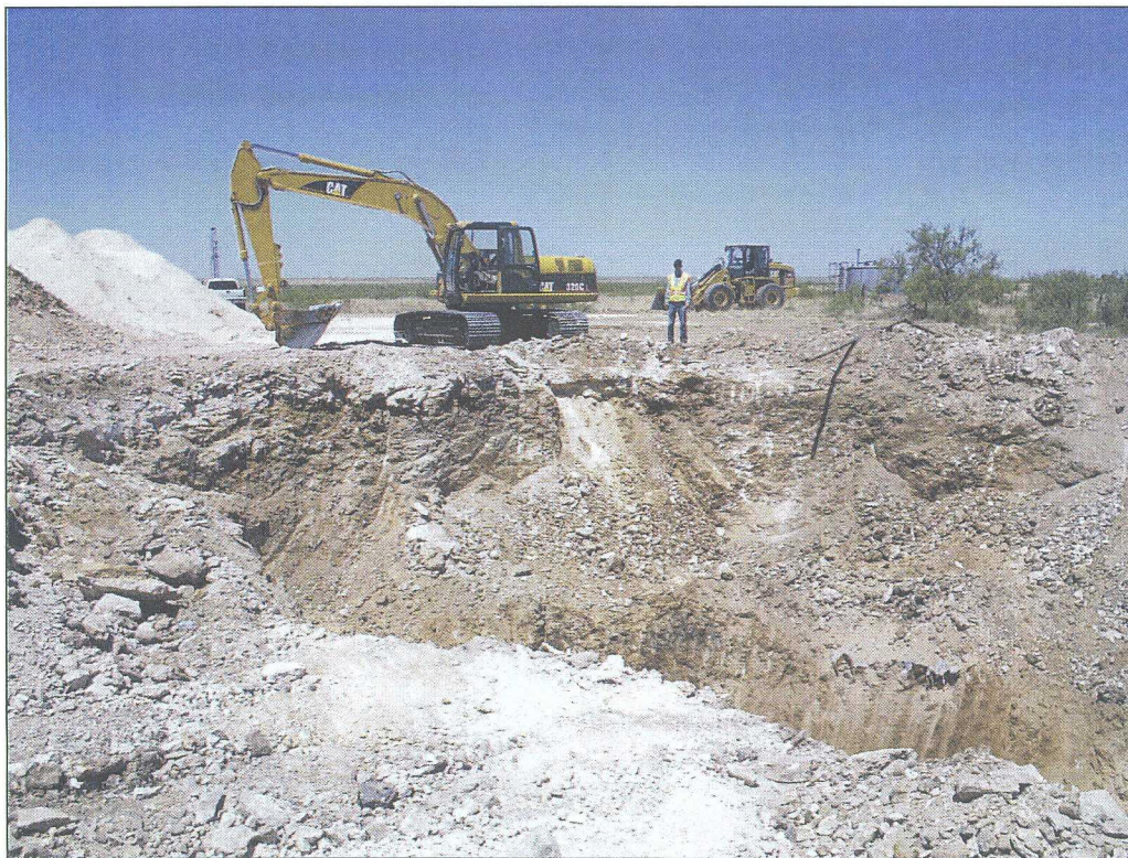
No. 8 – View to the west of the excavation after 1,400 cubic yards of contaminated soil had been removed off-site; photograph 1 of 3 (see Figure 5).
