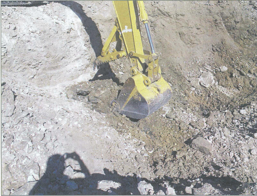
No 5 – View of the bottom of the excavation at 9 a.m. on June 11, 2008. A white/grey caliche layer is visible to the left of the photograph, while brown, sandy silt can be seen at the pit bottom.
