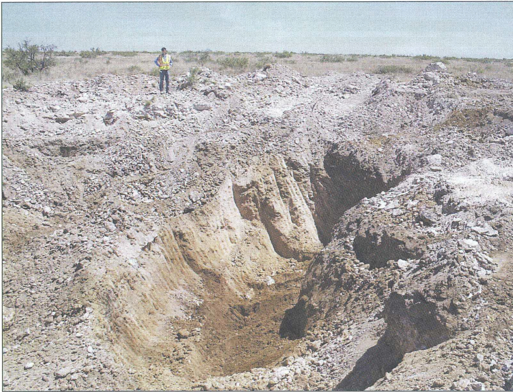
No. 7 – View to the north, northeast of the excavation after 1,400 cubic yards of contaminated soil had been removed off-site; photograph 2 of 2 (see Figure 5).
