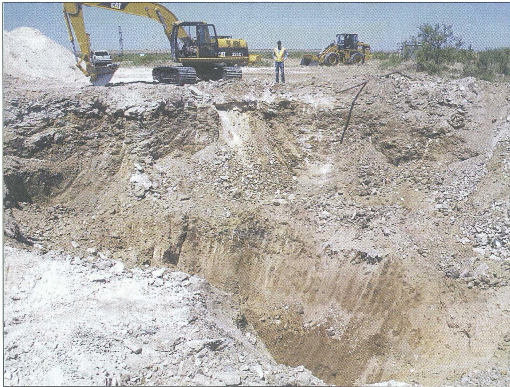
No. 10 – View to the west, southwest of the excavation after 1,400 cubic yards of contaminated soil had been removed off-site; photograph 3 of 3 (see Figure 5).
