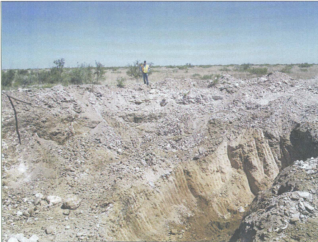
No. 6 – View to the north of the excavation after 1,400 cubic yards of contaminated soil had been removed off-site; photograph 1 of 2 (see Figure 5).
