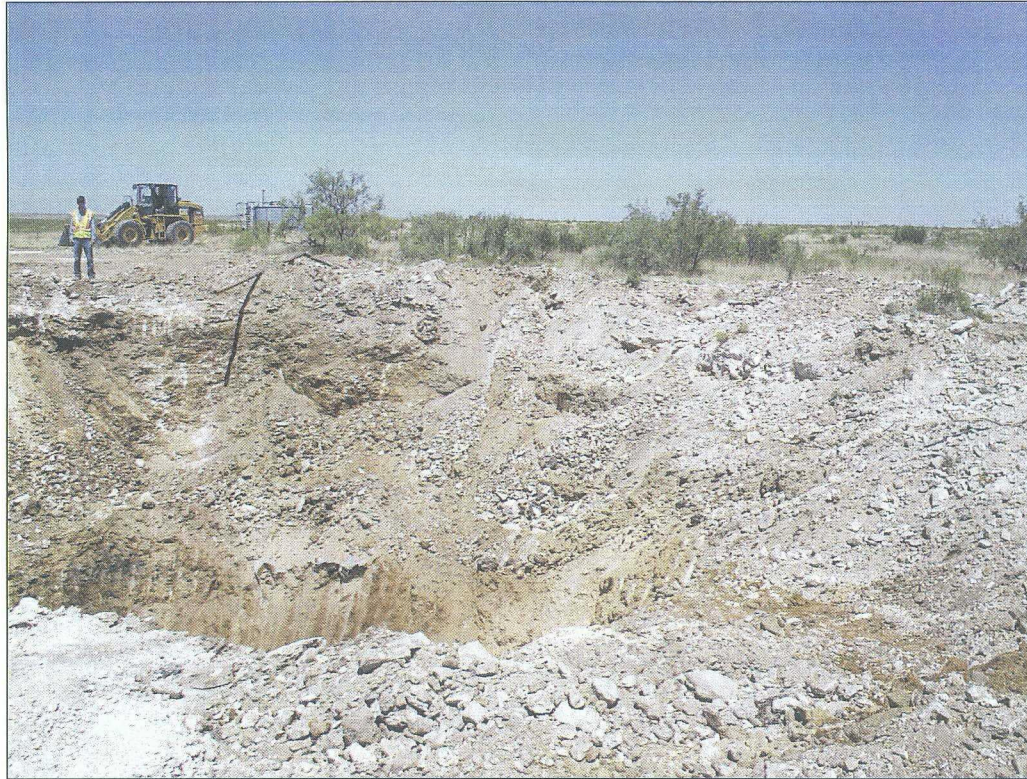
No. 9 – View to the northwest of the excavation after 1,400 cubic yards of contaminated soil had been removed off-site; photograph 2 of 3 (see Figure 5).
