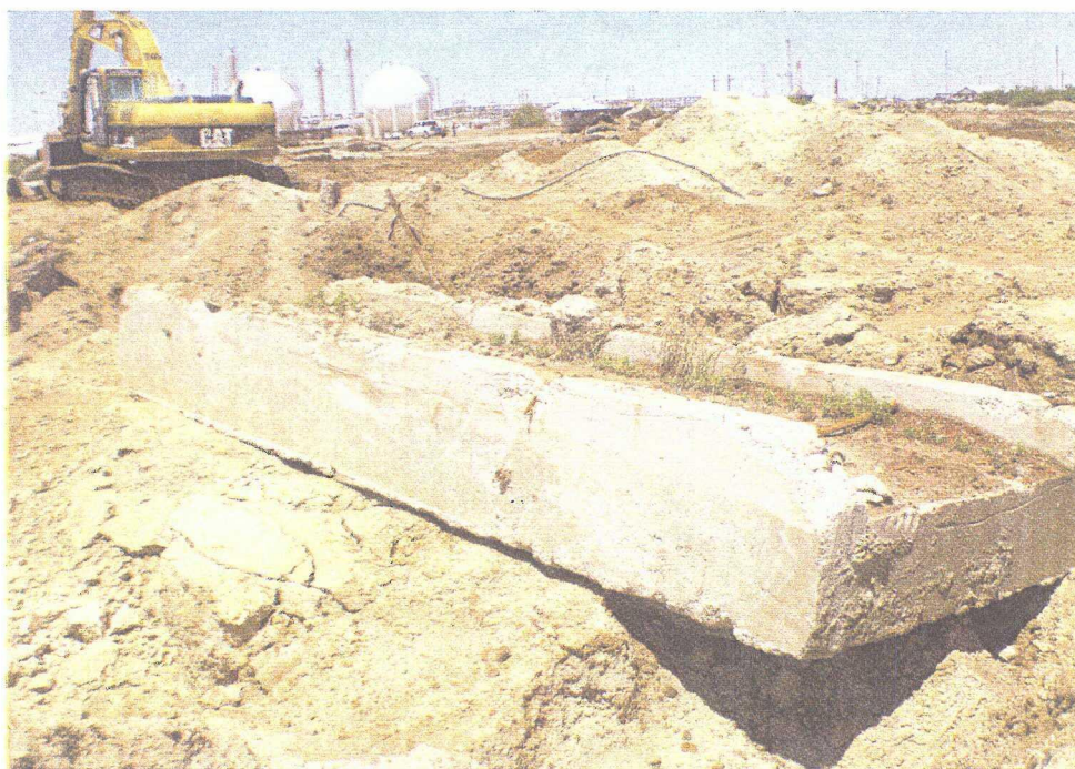
No 47 - This is one of three concrete slabs that are too heavy for the track hoe to load into the bin. It had to be left on site at central, Section E.
