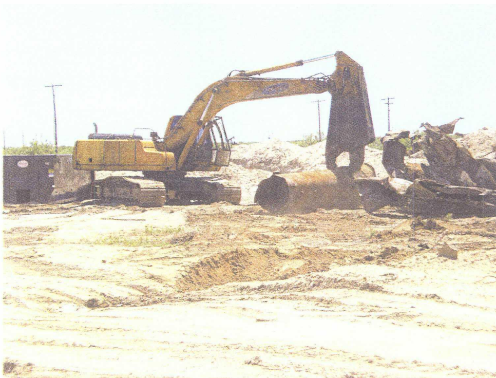
No 32 - This is in Section F, where the shears hoe was cutting pipe and large metal objects, such as vessels and pipe, into manageable lengths for loading into bins or onto flatbed trucks.
