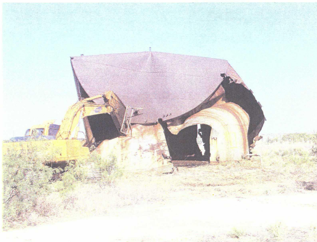
No. 7 – A hydraulic shear dismantled the tanks for recycling.
