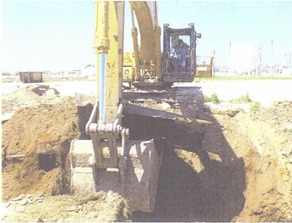
No 40 - This photo shows the removal of 1 of 2 septic tanks from the central area of Section H.
