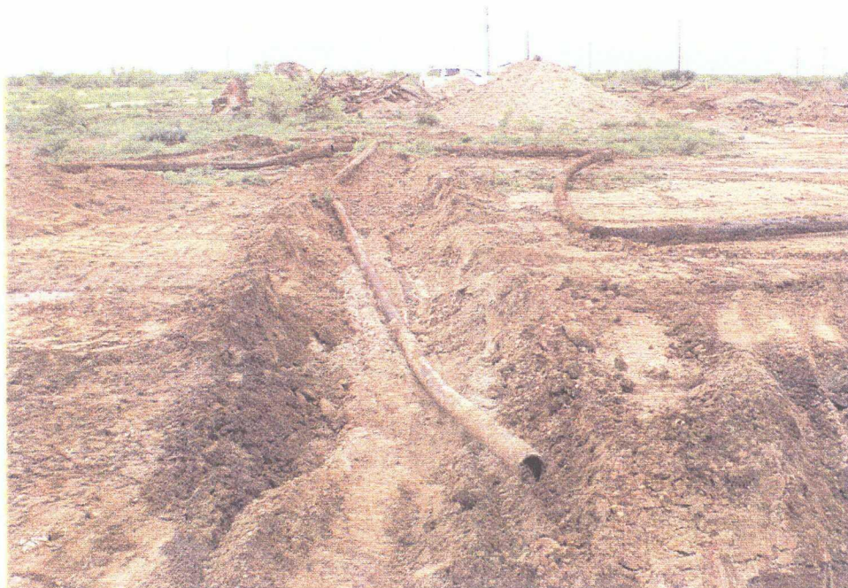
No 18 - This is Section C, looking south along a 5.5" pipe trench toward the pit of section D. The 7" pipe crosses the 5.5" at the bottom of the photo and is seen where it was pushed aside in the upper part of the photo.
