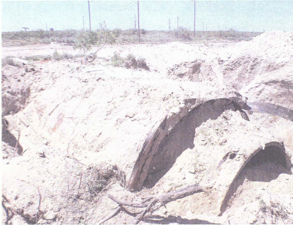
No 19 - This is D Section, looking north at the start of an excavation to pull up a large vessel. The vessel was buried in a pit that contained several smaller vessels as well as scrap metal and numerous pipe sizes and lengths. The pit took up a considerable portion of Section D.
