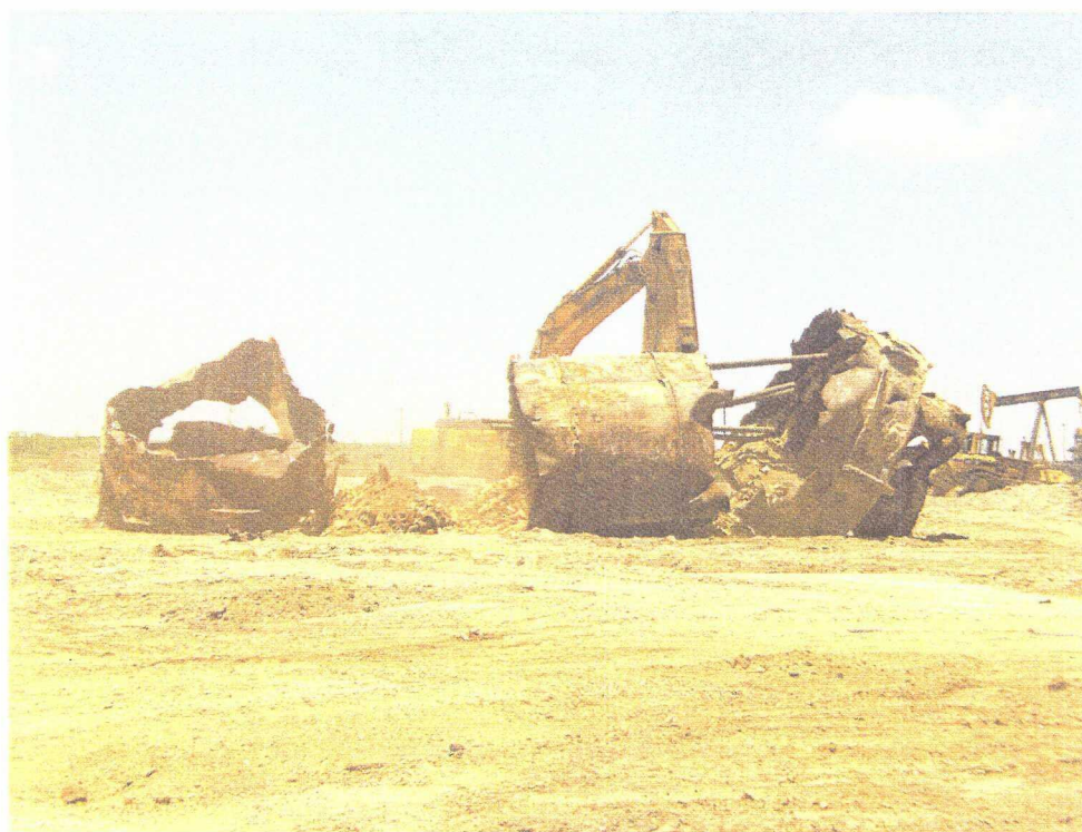
No 49 - This photo shows the shears hoe cutting apart the large vessel from Section D. The firebricks can be seen that formerly lined the vessel.
