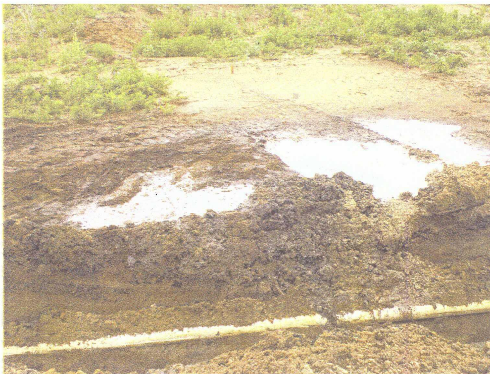
No 35 - This is another photo to demonstrate soil contamination. This is looking west in south-central Section B, at a surface, oily pool that is caving into a 2 ft. deep trench where 4" PVC is being excavated.
