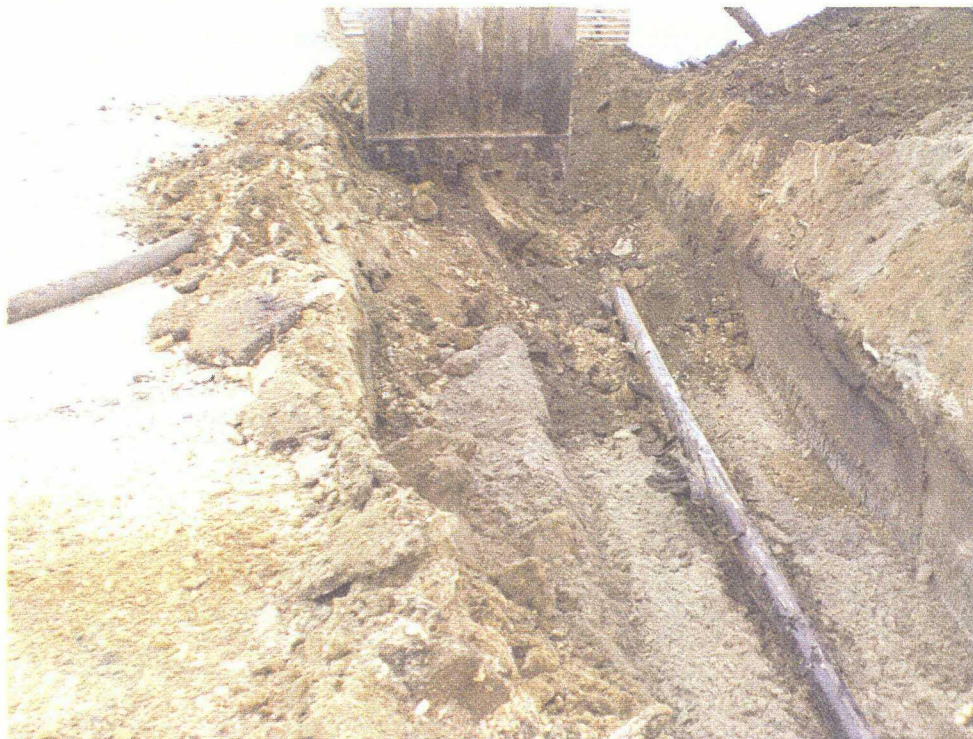
No. 26 – This is just north of central Section K, looking east along a trench where 3" pipe is being excavated at 3 ft.
