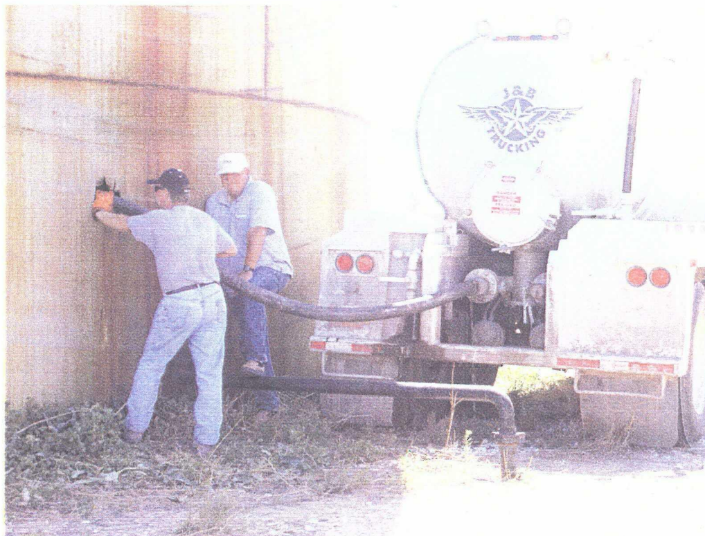
No. 5 – Vacuum trucks were used to remove flowable fluid from within the tanks.
