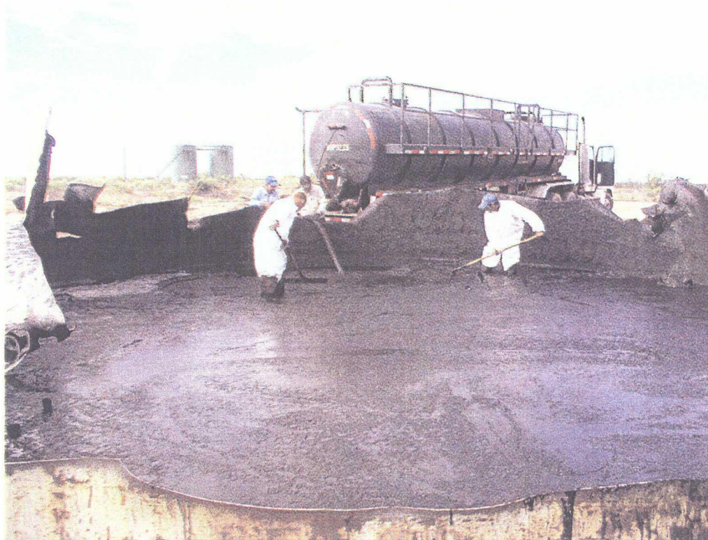
No. 11 – The tank bottom after all flowable material was removed from a tank, the shear tore the top of tank off so roustabouts could then push the thicker material to the vacuum truck for removal from tank.
