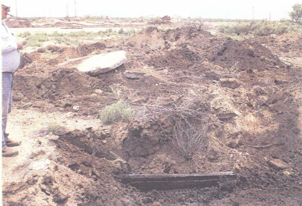
No 22 - This is Section G, looking southwest over an area from a north-central perspective. Concrete footings and a variety of pipe diameters and lengths were excavated in this vicinity. A 4" pipe is been excavated in the foreground.
