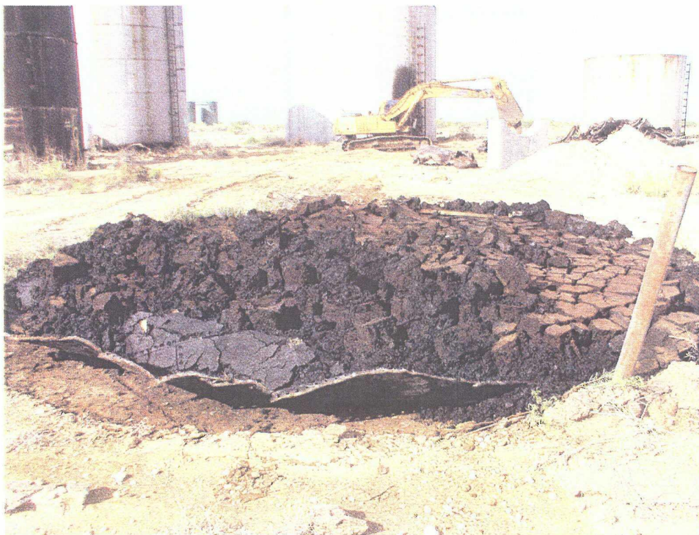
No. 10 – Non flowable sludge was loaded into covered roll offs for disposal.
