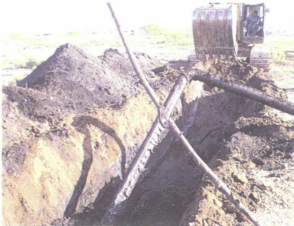
No 24 - This is Section I. The view is to the north where a 5.5" pipe-offset elbow is being pulled. Contaminated soils are clearly evident in the excavated materials.
