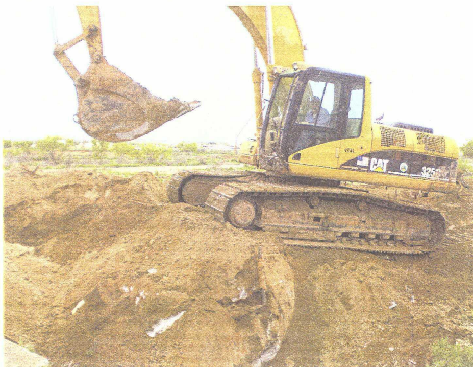
No 31 - This is the track hoe that was used to dig pipe, pull pipe, pull large objects from the pits, and to load trucks and bins. This photo was taken looking northwest from central Section E.
