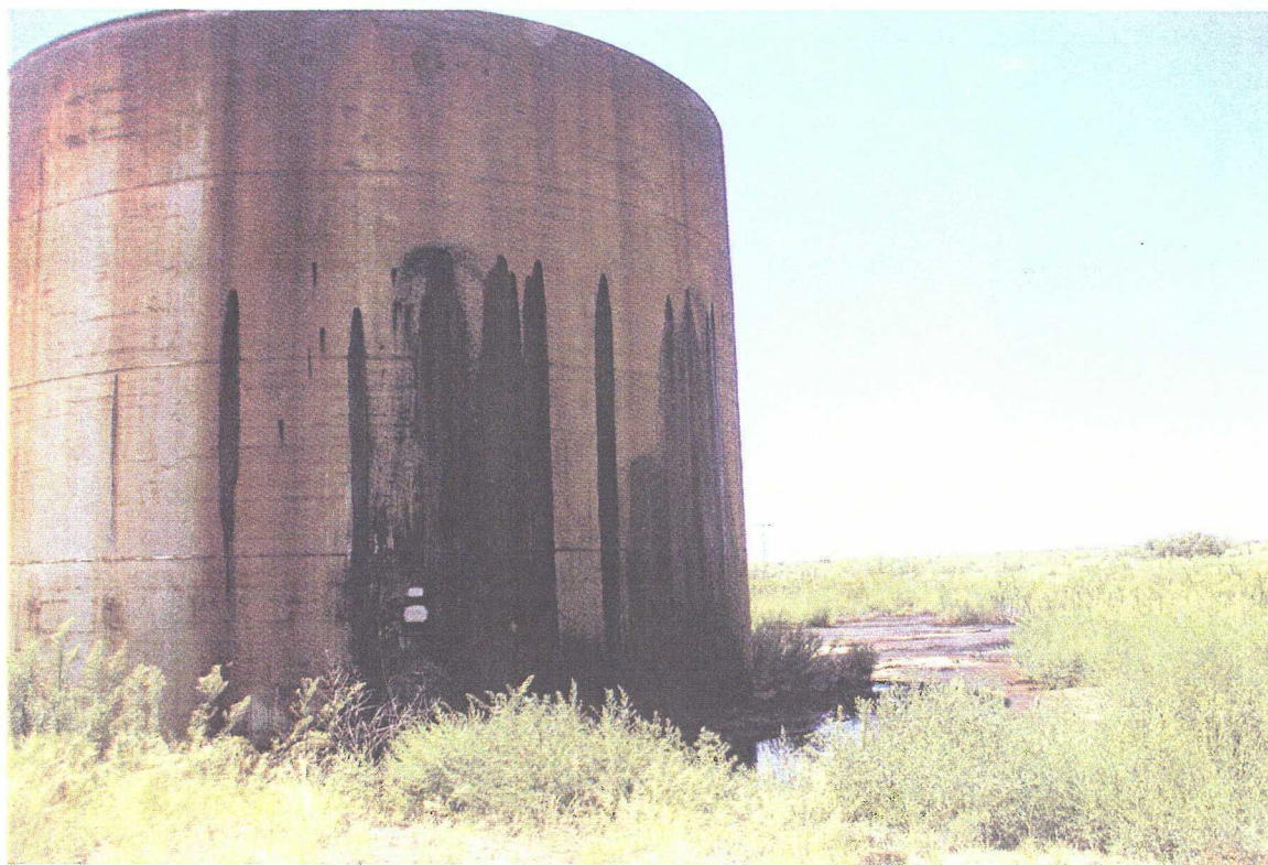
No. 3 – Some of the tanks had holes in them and crude oil leaked onto the ground as seen in the photograph.
