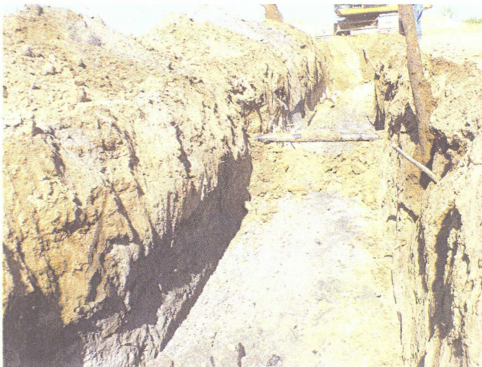
No 34 - This photo is to demonstrate contamination. It is looking west in the south of Section E, along a trench where 9" pipe is being excavated from 3.5 ft. The foreground shows a 4" pipe crossing. Soil discoloration and a distinct HC odor were observed from a depth of 2 ft.
