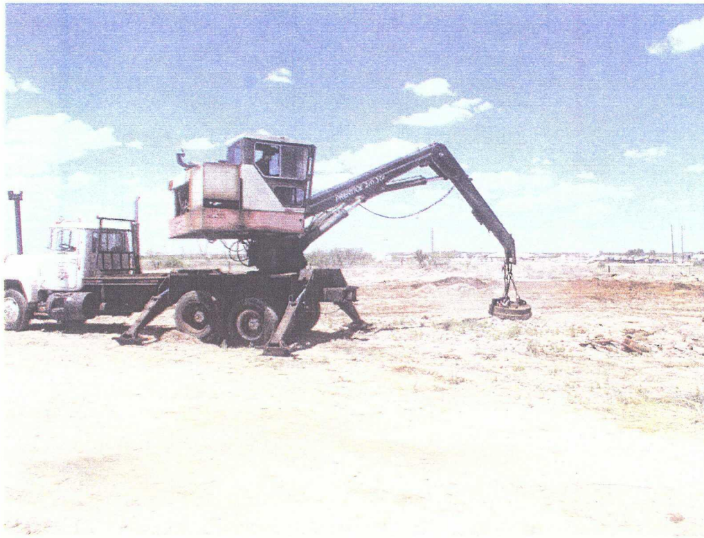
No. 13 – After completing the tank demolition and loading, an electric magnet went over the area to pick up the smaller pieces of steel for disposal.
