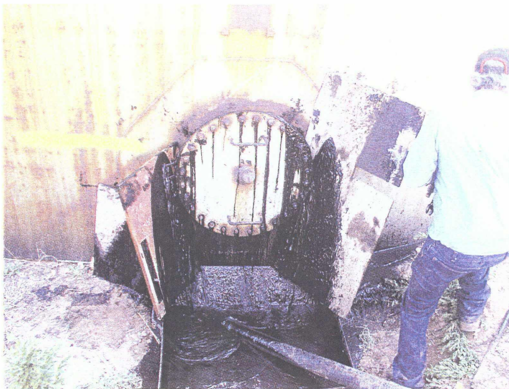
No. 6 – The man ways were carefully cracked open to access fluid when the valves on the tanks did not work. The vacuum truck pulled the fluid collected in the capture vessel.
