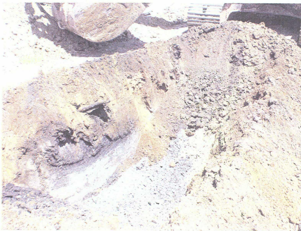
No 25 - This is Section J, looking to the northeast at a portion of 3" pipe trench which runs east-west. Soil discoloration can be seen to approximately 4 ft.
