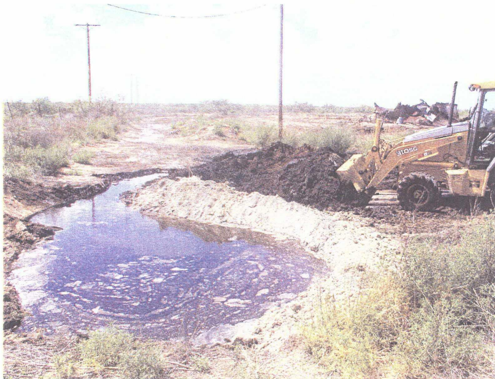
No. 14 – The sludge pile shown on Photo 2 was dug up and disposed of in the covered roll offs.
