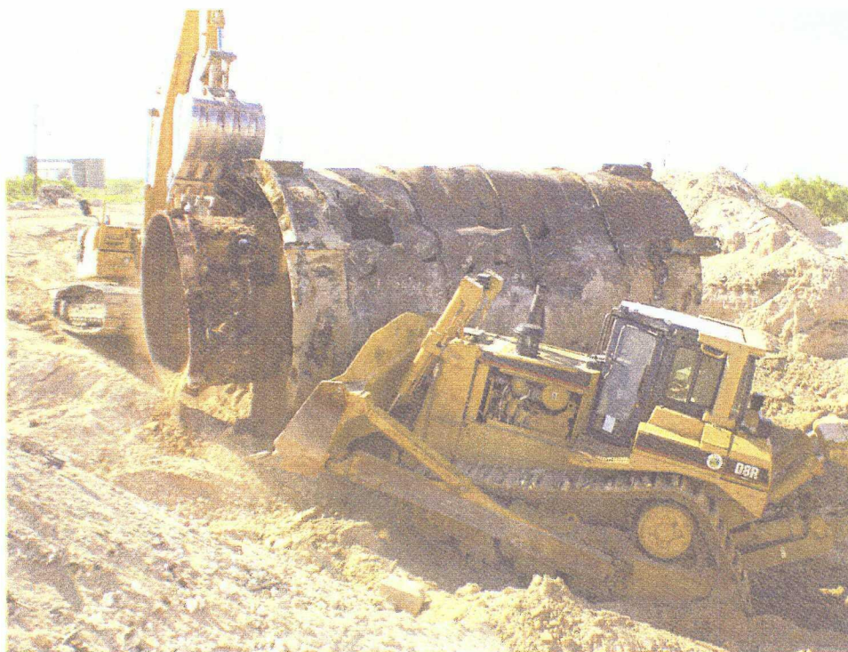
No 48 - This photo is of a D-9 Cat being assisted by the track hoe in extracting a large, brick-lined vessel from the pit in Section D. The D-9 was brought to site for this purpose. The track hoe was unable to budge the vessel under its own power.
