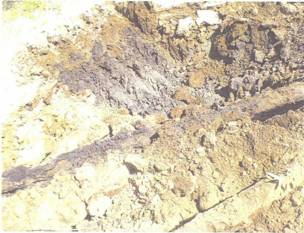
No 28 - This is Section M, looking southeast at two shallow 3" pipes that were dug out of some shallow, discolored soils.
