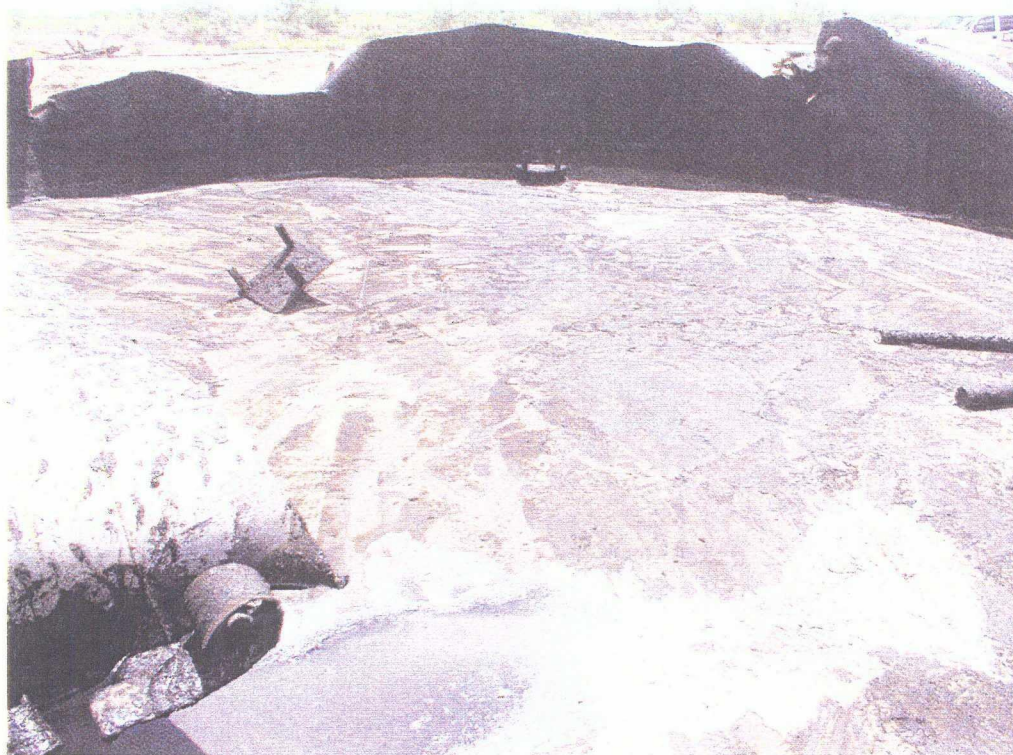
No. 12 – The tank bottom after the roustabouts finished cleaning out fluid.
