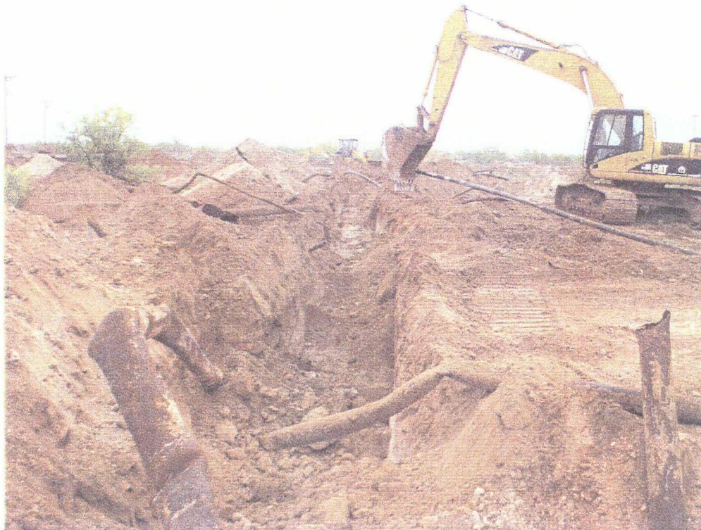
No 21- This is Section F, looking south into a trench containing 5.5", 4", and 3" pipe.
