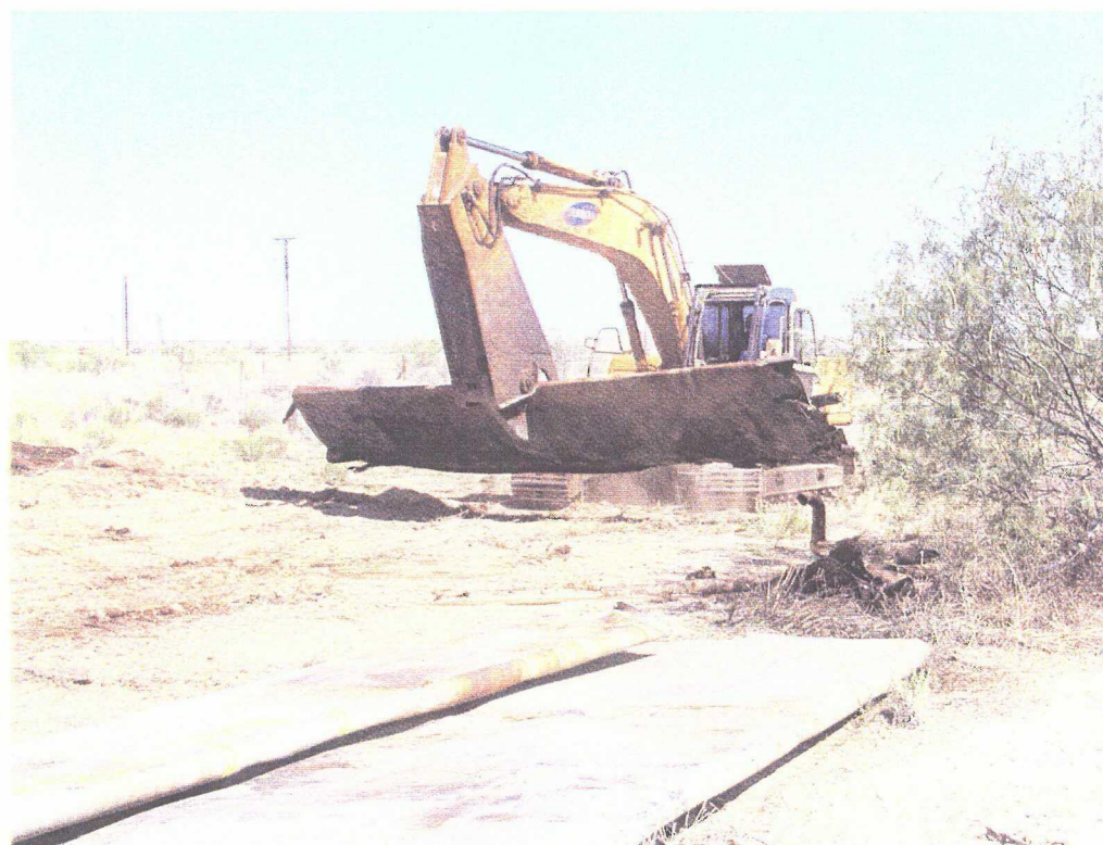
No. 8 – The sheared tanks were folded up for transport offsite.
