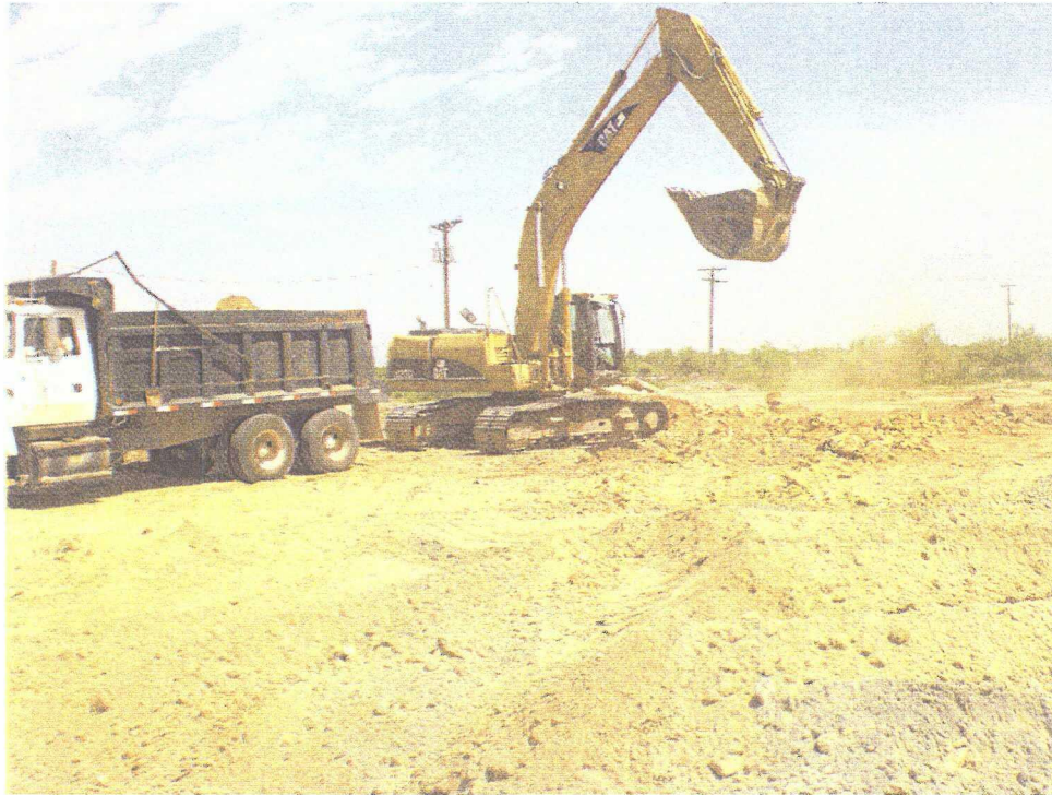
No 50 - This photo shows the track hoe loading firebricks onto the dump truck.
