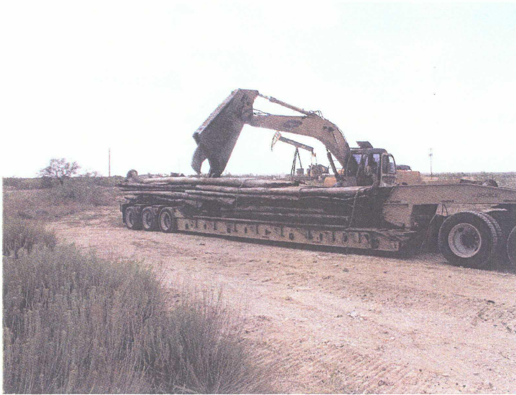
No. 9 – The folded up steel loaded on trucks for transport offsite.
