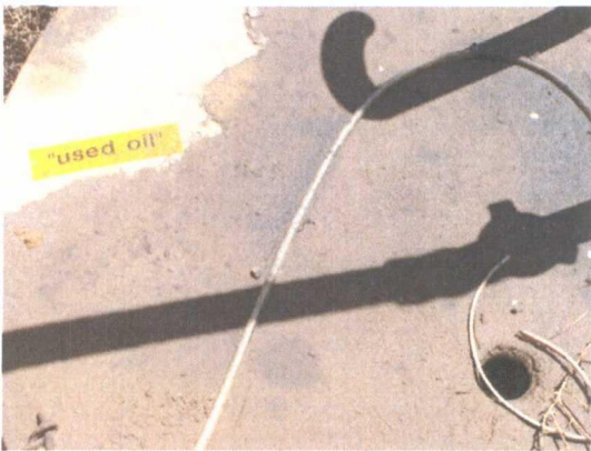
Photo 7: Port with missing lid on BGT.
