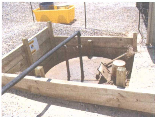
Photo 5: BGT with hatch open but covered with 5 gallon can.
