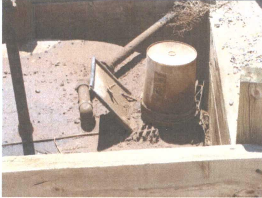
Photo 6: 5 gallon can over hatch of BGT.
