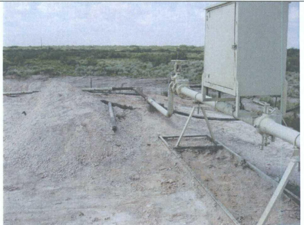
7-13-07 RMA excavated contaminated soil from around piping
