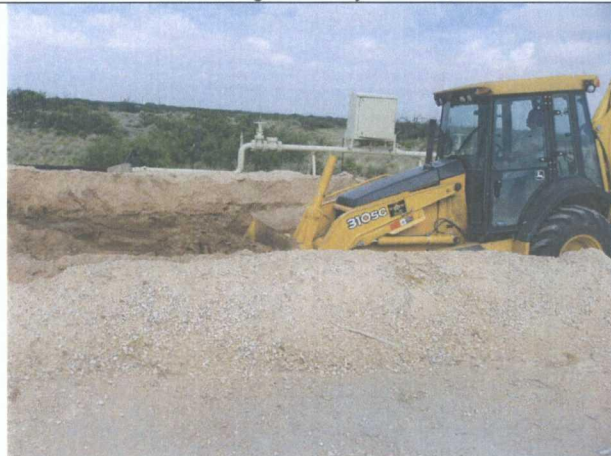
8-1-07 second excavation on elevated areas according to analytical data. Excavated approximately 6 feet in firewall area
