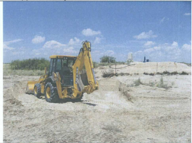
8-1-07 second excavation on elevated areas according to analytical data. Excavated approximately 3 additional feet in area south of firewall across fence
