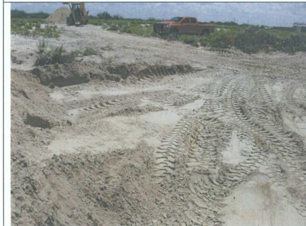
8-1-07 second excavation on elevated areas according to analytical data. Excavated approximately 3 additional feet in area south of firewall across fence
