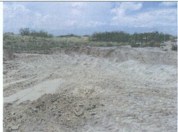
8-1-07 second excavation on elevated areas according to analytical data. Excavated approximately 3 additional feet in area south of firewall across fence
