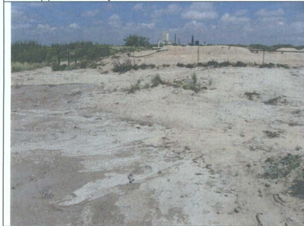
8-1-07 second excavation on elevated areas according to analytical data. Excavated approximately 3 additional feet in area south of firewall across fence
