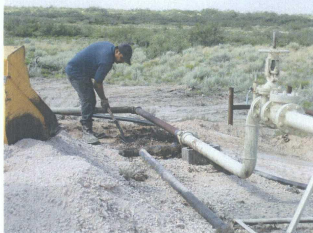
7-13-07 RMA employees removing contaminated soil from around piping
