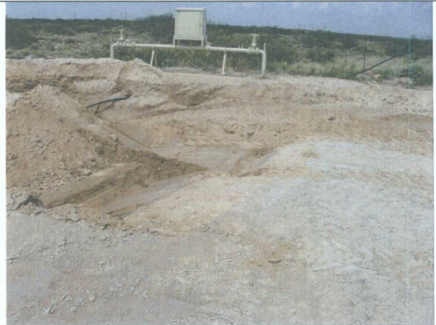
8-1-07 second excavation on elevated areas according to analytical data. Excavated approximately 3 feet in area north of firewall
