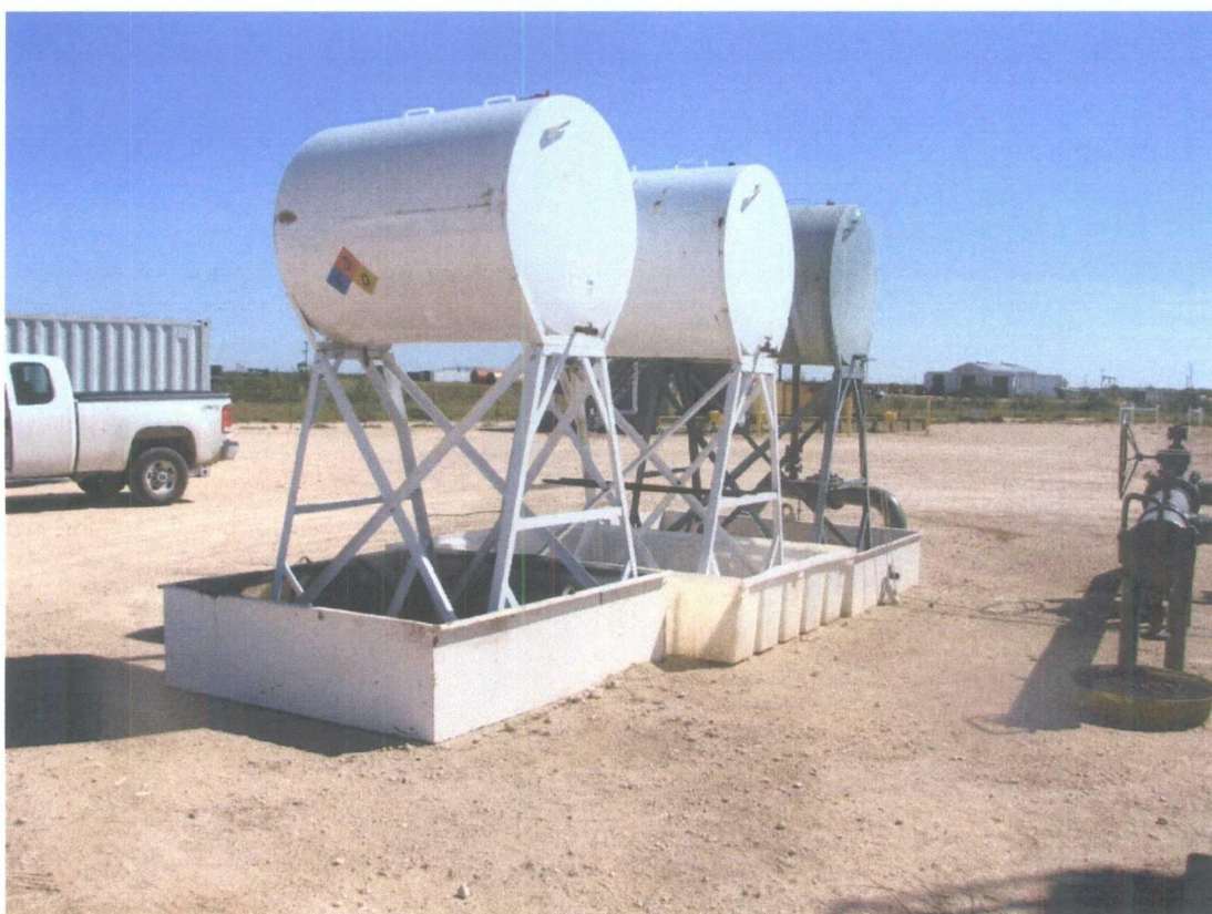
Photos Taken 10/10/08 After containment was installed
